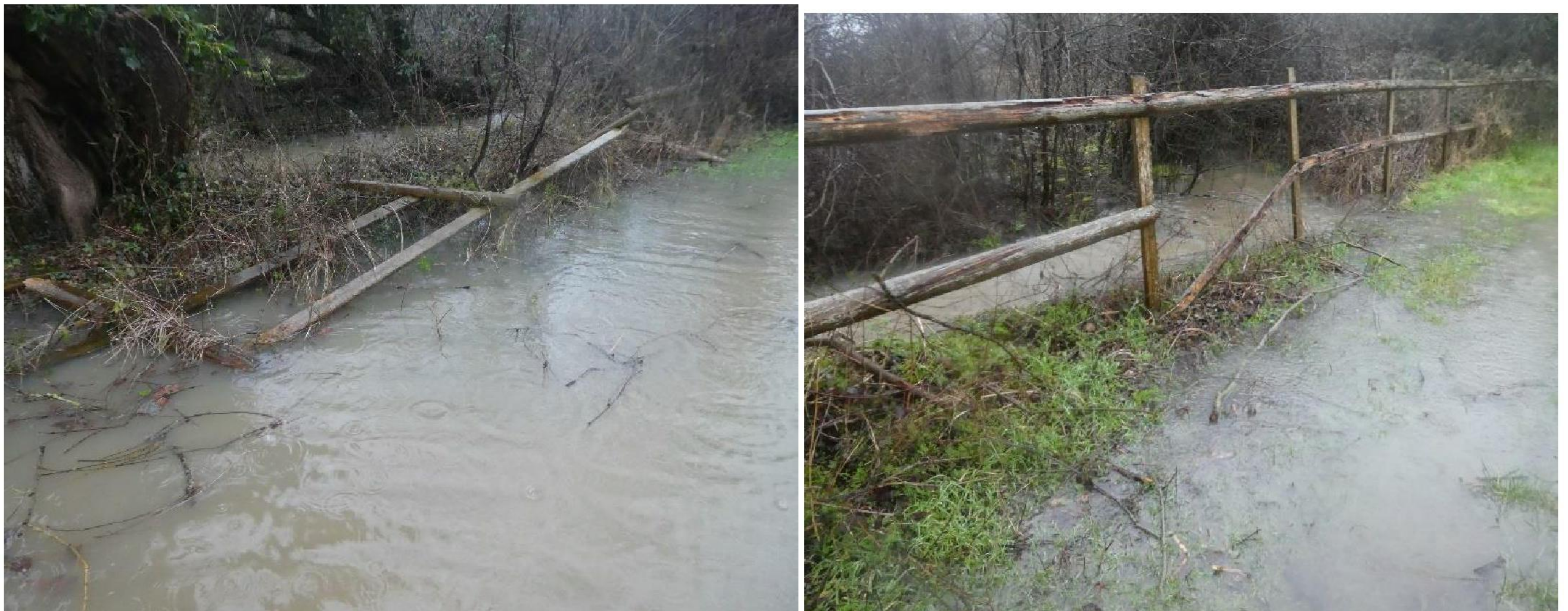
C – Flooded stream east of the bridge which is overflowing onto the footpath 27/01/2026 11:20am
