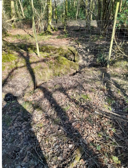
View of discharging ditch immediately north of existing pond, in northwest corner of Field 8/Hurst Farm. Ditch shown to be directed into east to west ditch located adjacent to site's northern boundary.
