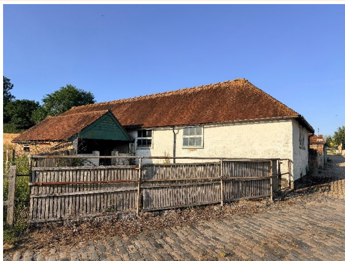
Photograph 1. Western elevations of the main stable and adjoining stable.
