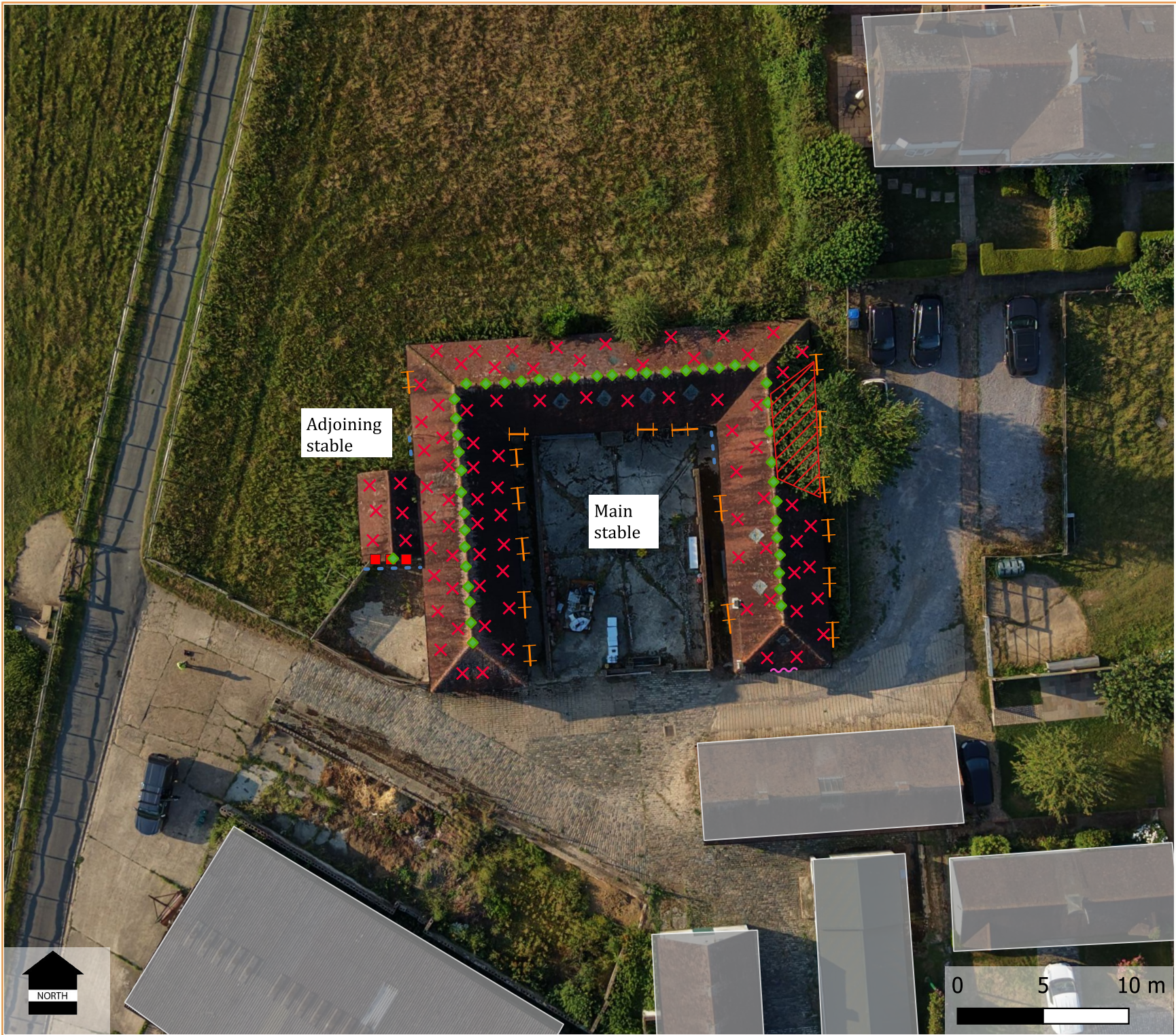
Figure 2. Results of the external building inspection
