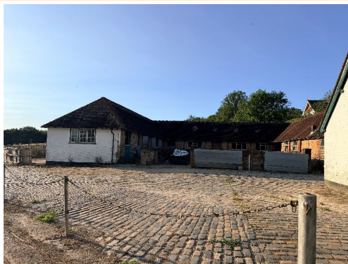
Photograph 2. Southern elevation of the main stable.
