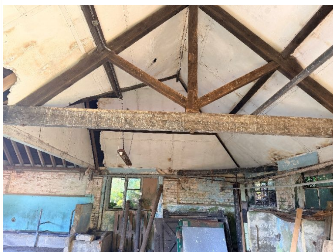
Photograph 5. Internal view of the northeastern section of the main stable, showing the wooden boarding.
