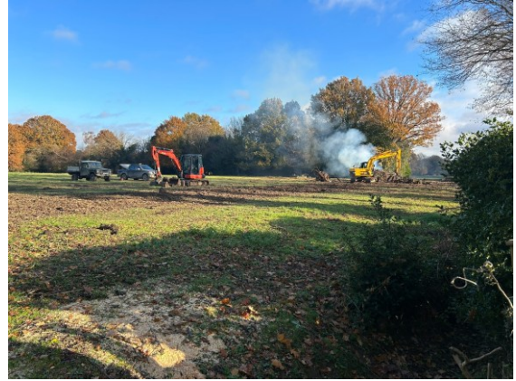
P16 | 23 November 2023 – vehicles and machinery clearing trees and hedgerows.
