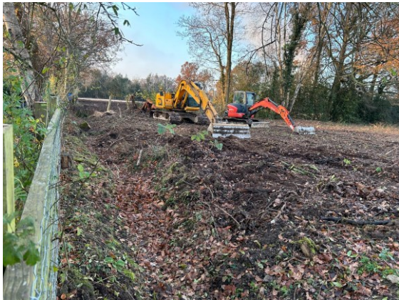
P17 | 1 December 2023 – hedgerow clearance along an alignment which appears consistent with the proposed perimeter road; Council should verify against the submitted plans.
