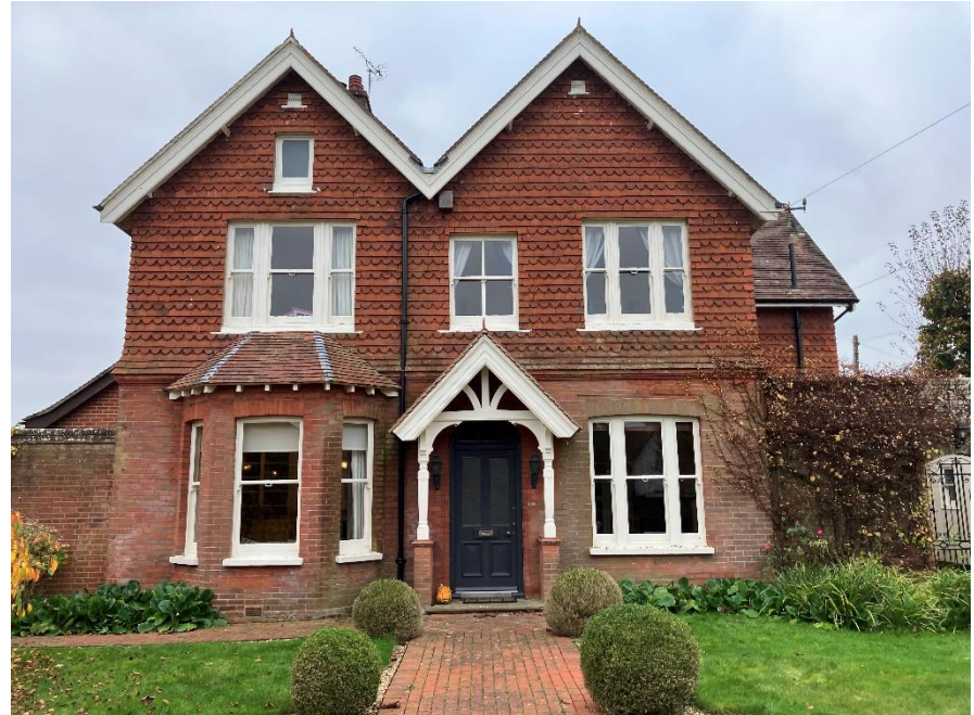
Photo 5: Front Elevation facing towards Hassocks Road, although unfortunately largely hidden from view.
