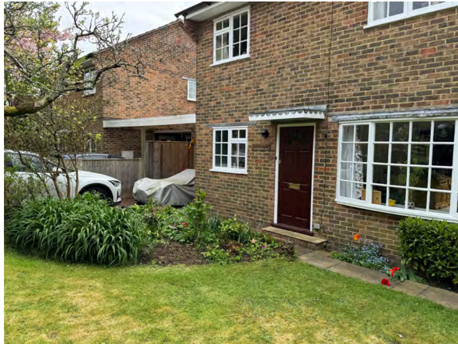
View of existing front entrance, car port between properties (to be demolished) and lounge bay window - the location for the single storey extension
