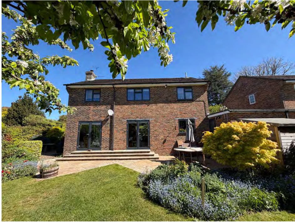
View of rear (south-west) of 3 Hobdens Lane
