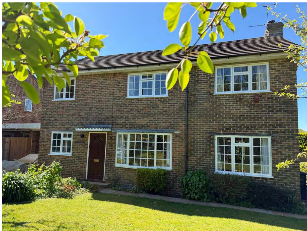
View of front elevation facing north-east
