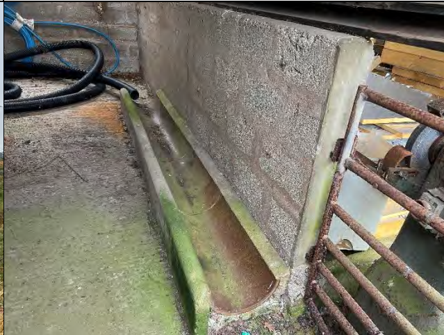
Fibrous guttering in the north-east of the building.
