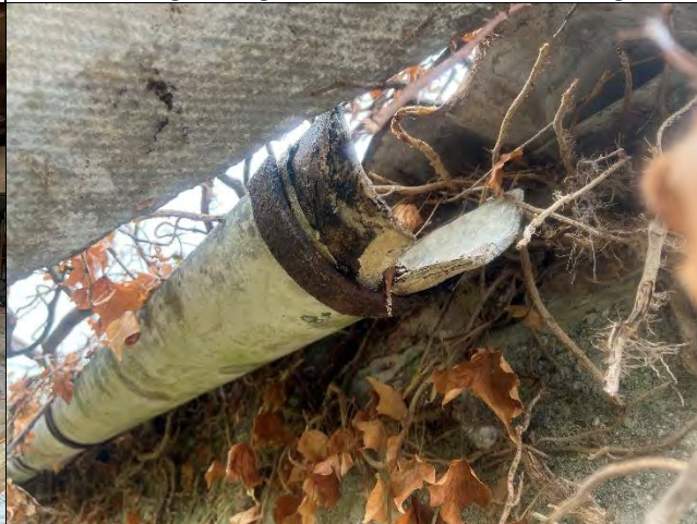
Fibrous guttering in the north-east of the building.
