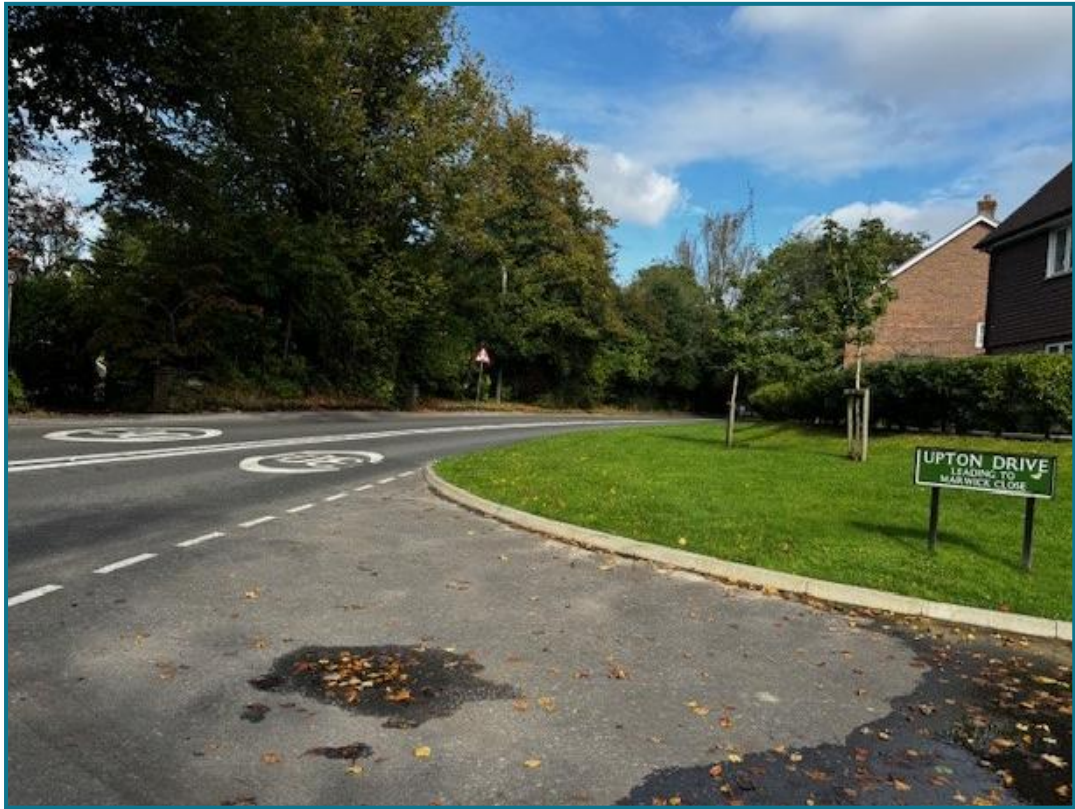
Figure 2.1 – Eastbound visibility from Upton Drive / A272
