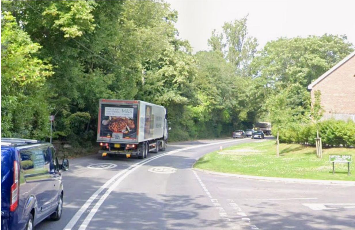
Figure 2.2 – View looking eastbound along A272 showing narrow carriageway lanes and narrow footway.
