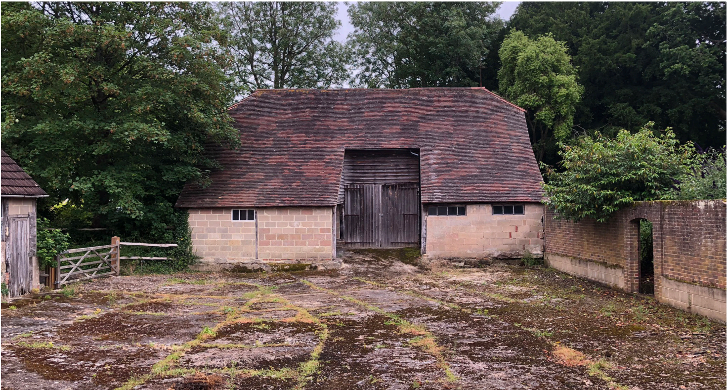
The Barn, with modern blockwork repairs
