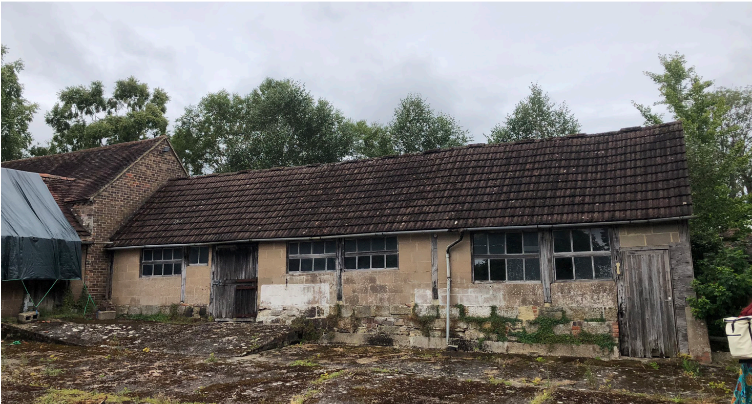
The Stables, with modern concrete tiles and blockwork
