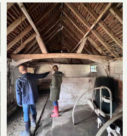
QUEEN POST TRUSS ROOF SYSTEM
