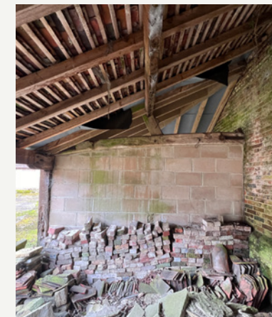
BLOCKWORK, RAFTERS AND BRICK WALL
