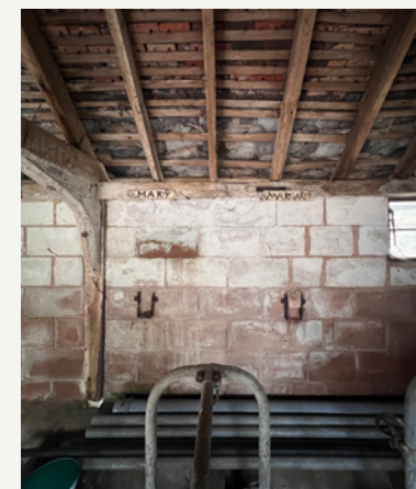
BLOCKWORK AND RAFTERS
