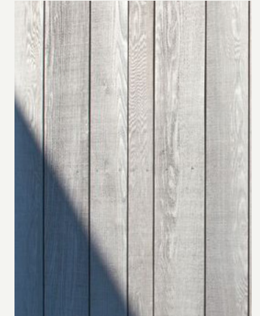
WIDE FORMAT VERTICAL TIMBER BOARDING
