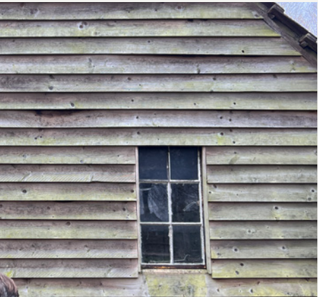
Stables & barn: horizontal timber weatherboarding
