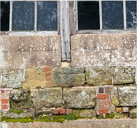
Stables: Brick & Stone plinth with timber post
