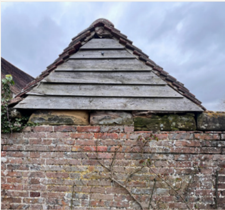
Brick Garden Wall + Cow-Shed Gable
