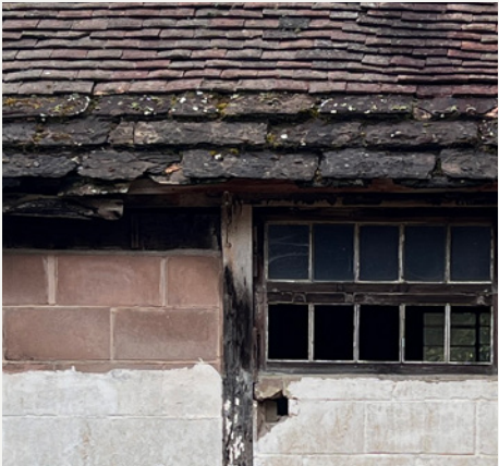
Cow Shed: Perimeter stone and clay roof tiles with timber and concrete block below
