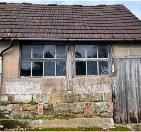
Stables: Modern block infill above plinth with modern roof tiles and rainwater goods
