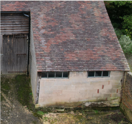
Barn: Tiled roof with modern infill blockwork to west facing elevations. Vertical timber entrance doors ledged and braced internally
