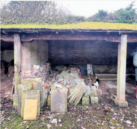
Byre: Brick rear wall, modern concrete block infill, timber post and staddle stone to facade, weather clay tile roof
