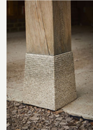
STADDLE STONE DETAIL: REFURBISHED WHERE SUITABLE
