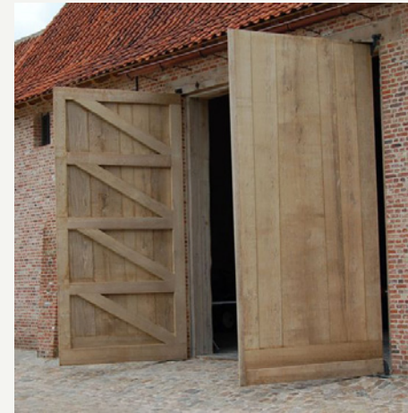
LARGE TIMBER BRACED DOORS THE BYRE
