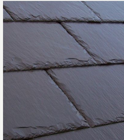
NATURAL SLATE TILE ROOF THE STABLES
