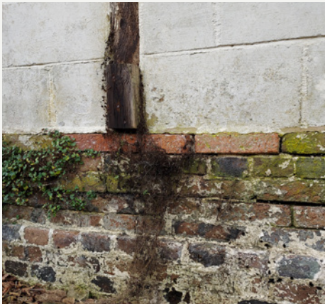
Cow Shed: Brick plinth with timber post and concrete block infill
