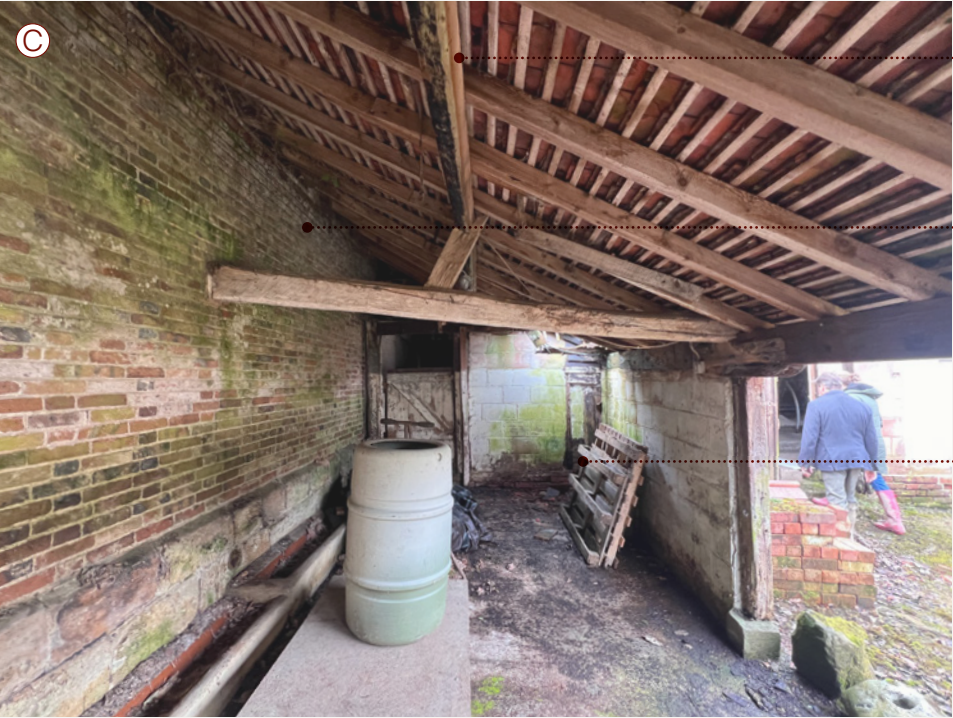
G03 - BYRE LOOKING WEST
