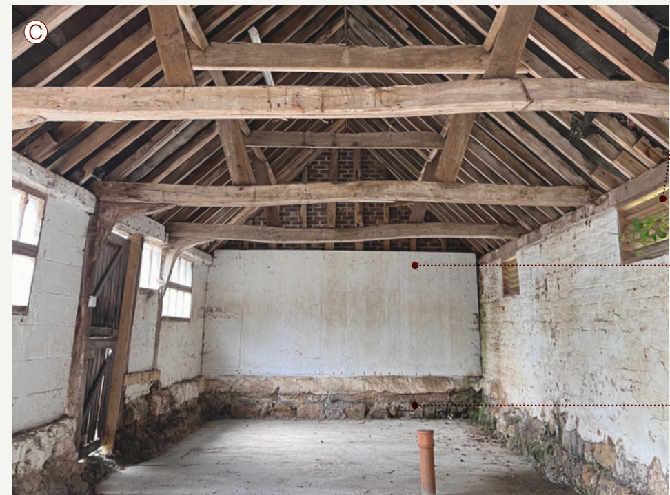
G15 - STABLES ROOM 1
