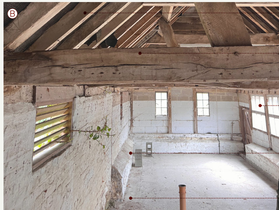
G17 - STABLES ROOM 2
