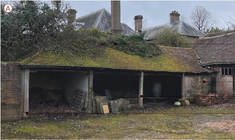
BYRE - VIEW FROM NORTH-EAST
