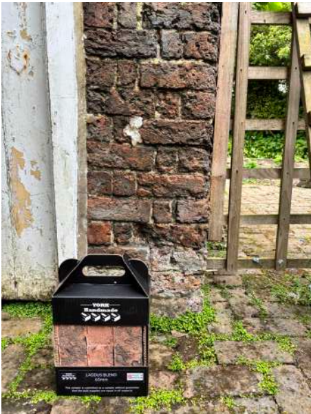
York Handmade Laddus Blend 215mm x 65mm x 102.5mm in flemish bond
