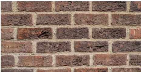
York Handmade Laddus Blend 215mm x 65mm x 102.5mm in flemish bond
