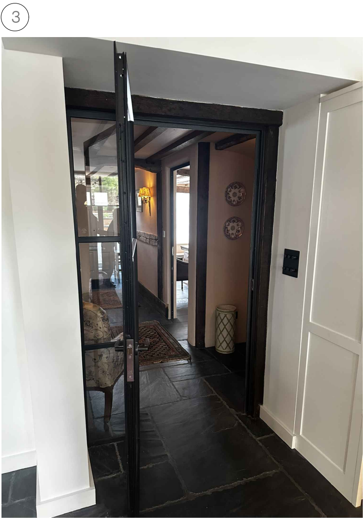
New crittle style door between existing dwelling and new extension
