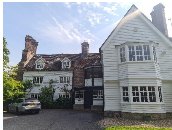
Plate 1. Northern elevation of Building B1 (NE section)
