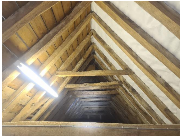
Plate 7. Timber frames in main loft void
