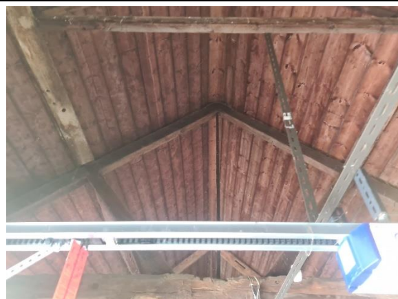
Plate 18. Internal view of B4
