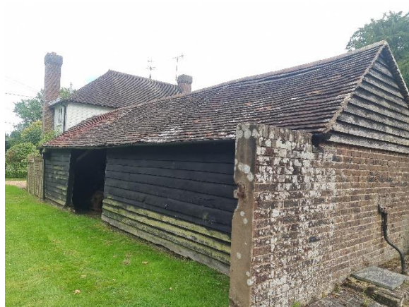
Plate 15. Outbuilding B3 – north-west aspect
