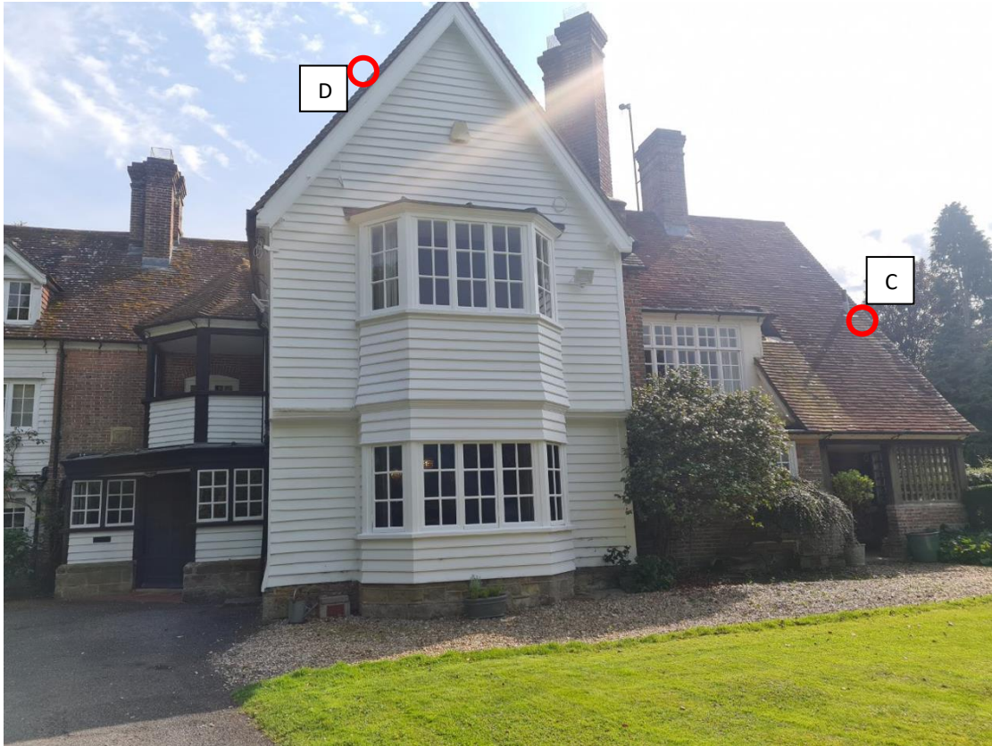
Image 3 – The emergence point of 1 x common pipistrelle (C) from a roof tile on the north-west corner of Building B1 on 01.08.24; and 1 x brown long-eared bat (D) from near the ridge of the roof on the northern extension on 22.08.24
