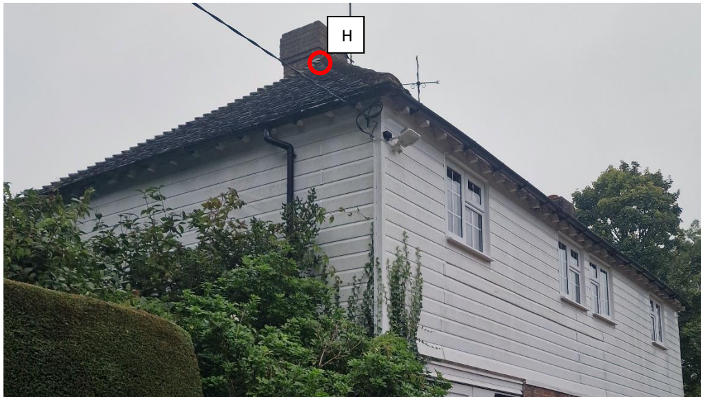
Image 4 – The emergence point of 3 x common pipistrelles from a roof tile beneath the chimney on the southern elevation of Building B2
