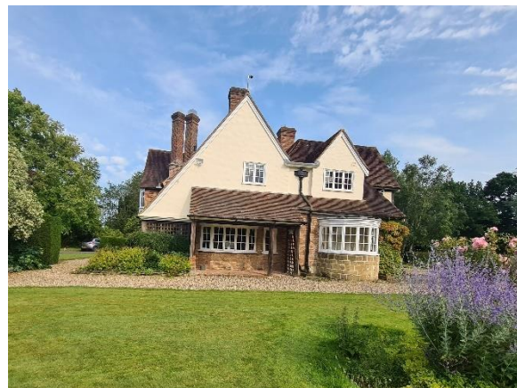
Plate 3. Western elevation of Building B1
