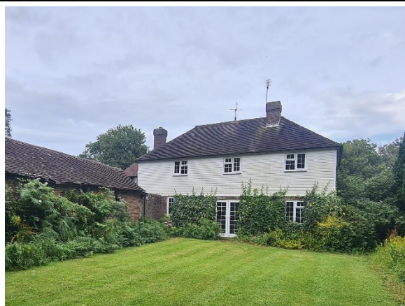
Plate 11. Western elevation of Building B2
