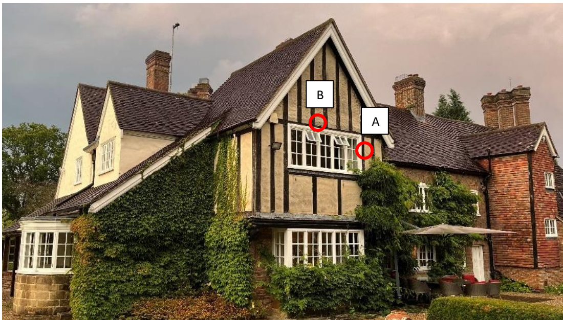
Image 2 – The emergence point of 8 x soprano pipistrelle (A) and 1 x common pipistrelle (B) from a gap in the wall between the timber frame and wattle-and-daub composite to the right of a second-storey window on the southern elevation of Building B1
