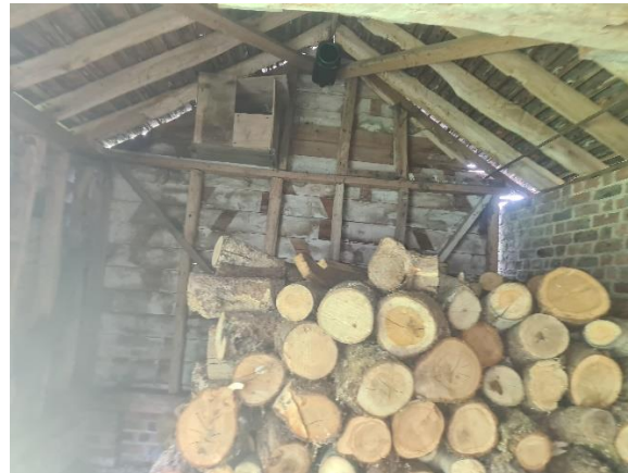
Plate 16. Internal view of B3
