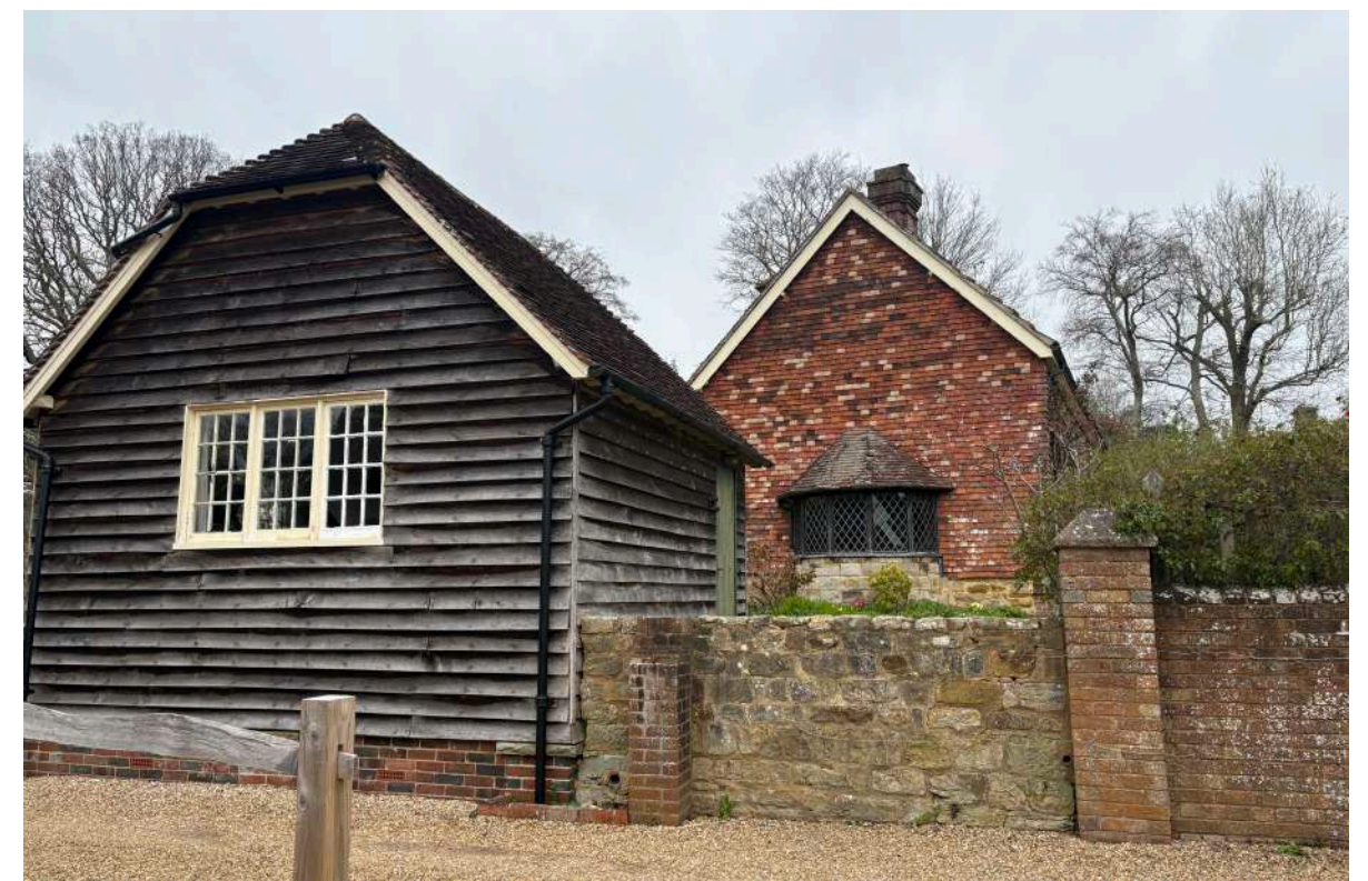
Daltons Farm from the south (access to The Byre and the application site). The former granary is in the foreground
