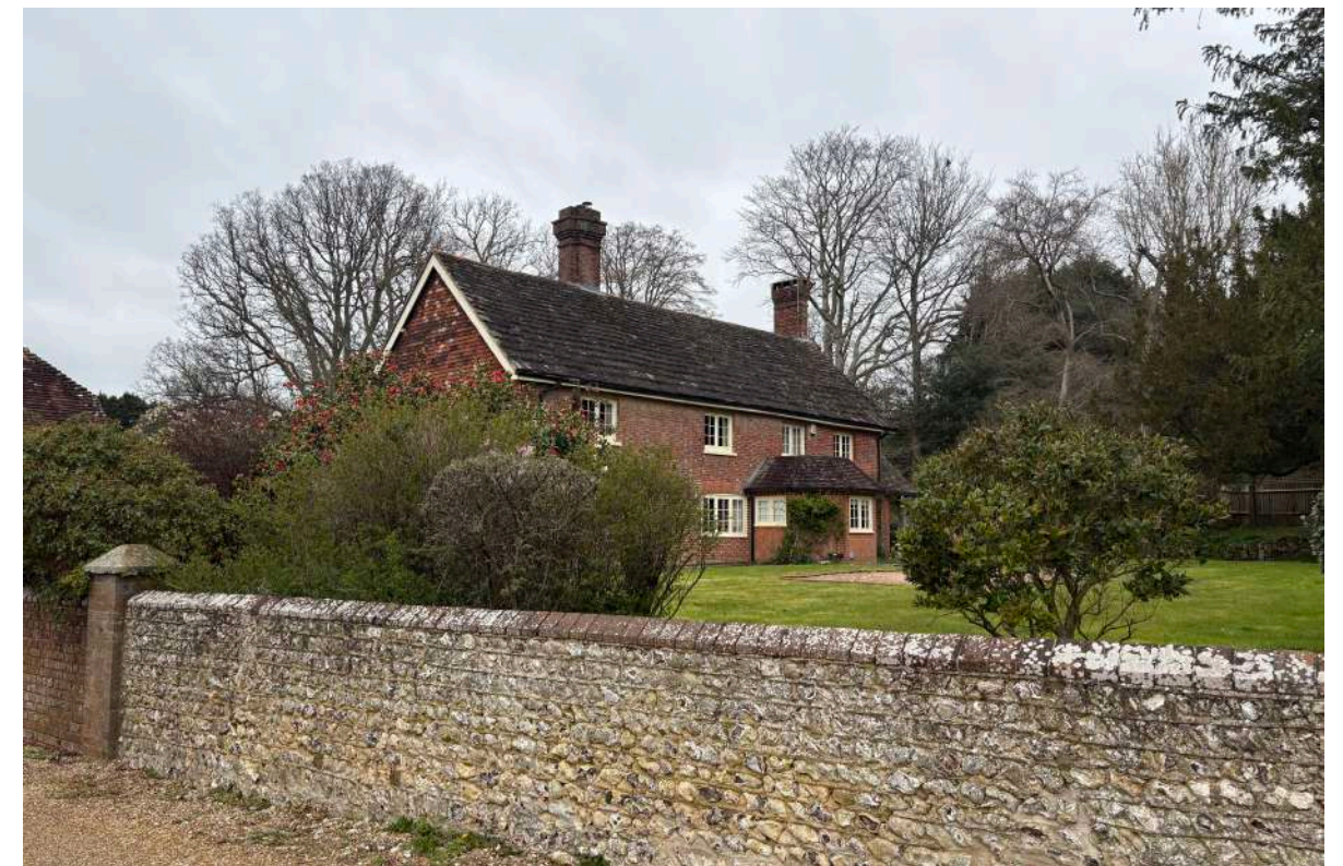
View north-west towards Daltons Farm from The Street. Its primary elevation and walled grounds are shown
