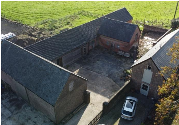
Figure 1 – Existing south elevation
