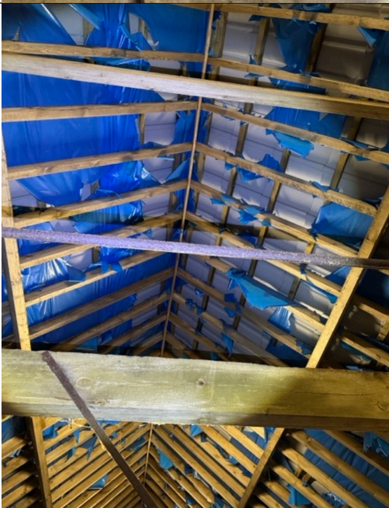
Photograph 10: The roof structure of the barn section B
