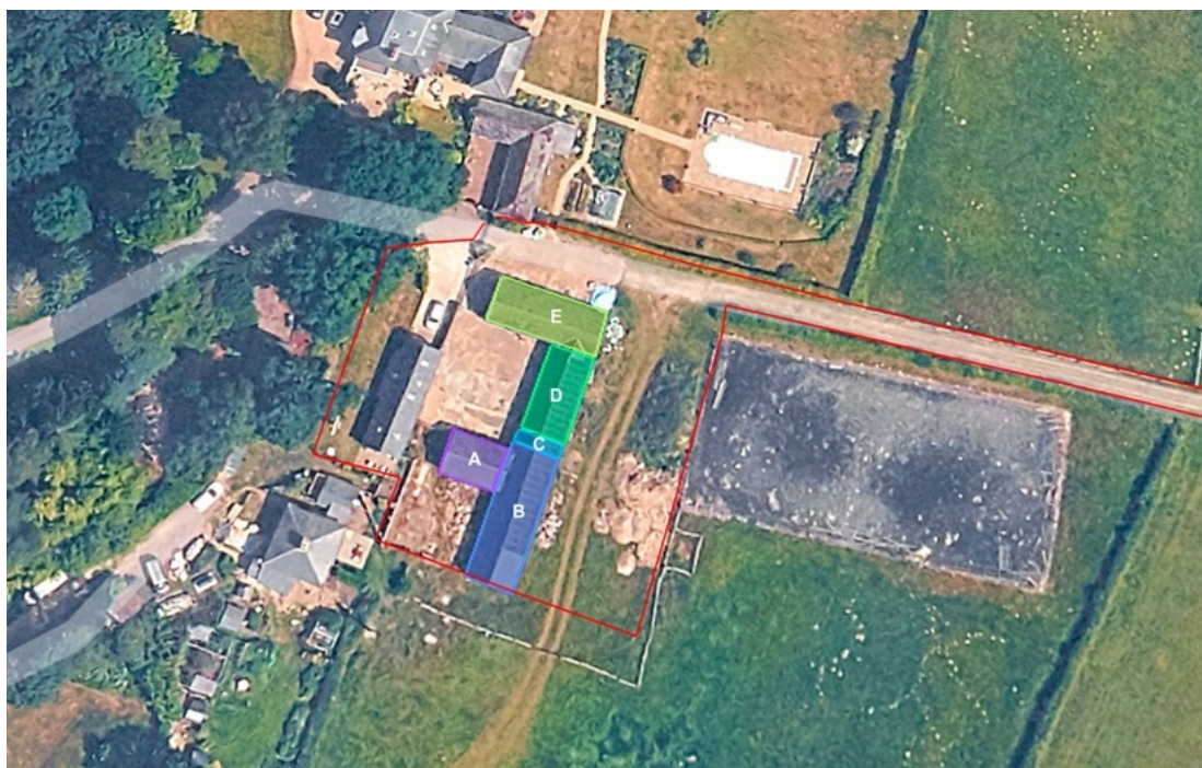
Figure 3: The remaining barns which are to be converted under the application
