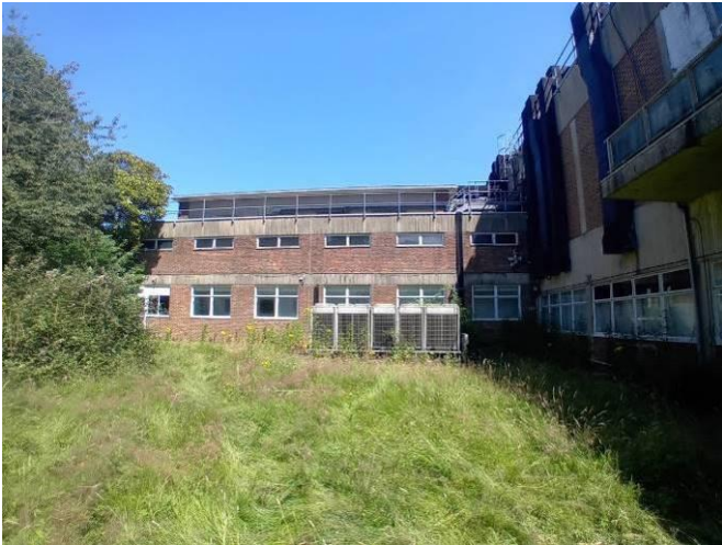
Plate 27: Area to the rear of the EDF Energy building – location of WLS110.
