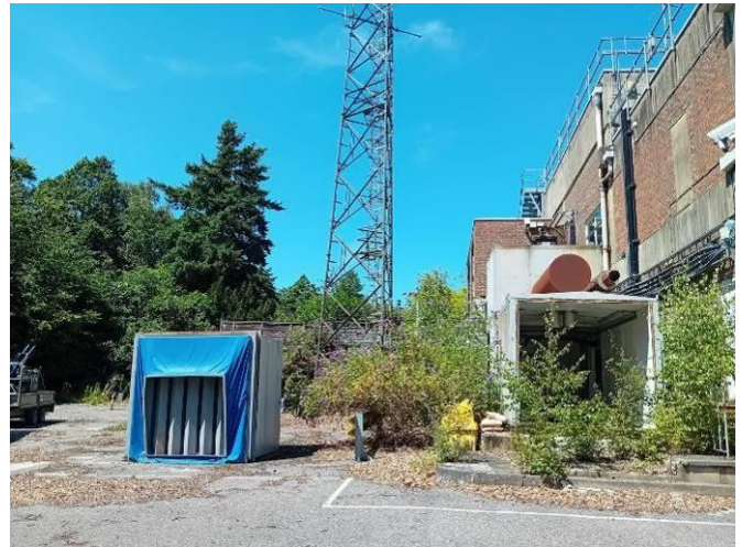
Plate 22: Generator building, telecommunications mast and other infrastructure to the rear of the EDF Energy building.
