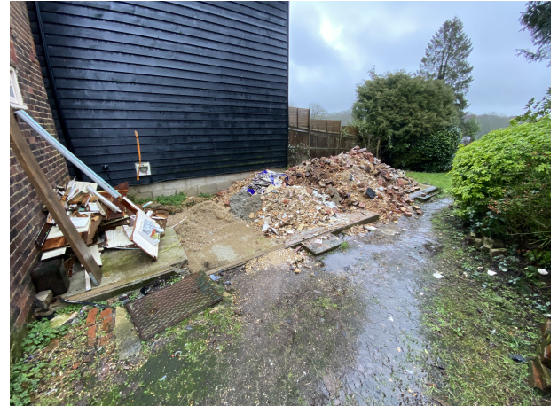
Photo of the existing concrete pads to the rear of the property
