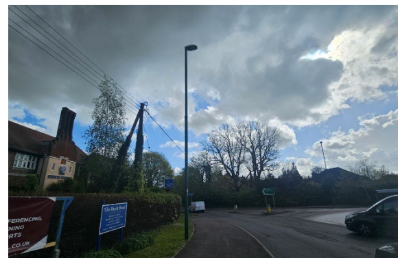
Figure 2: The entry to the west end of the Conservation Area
