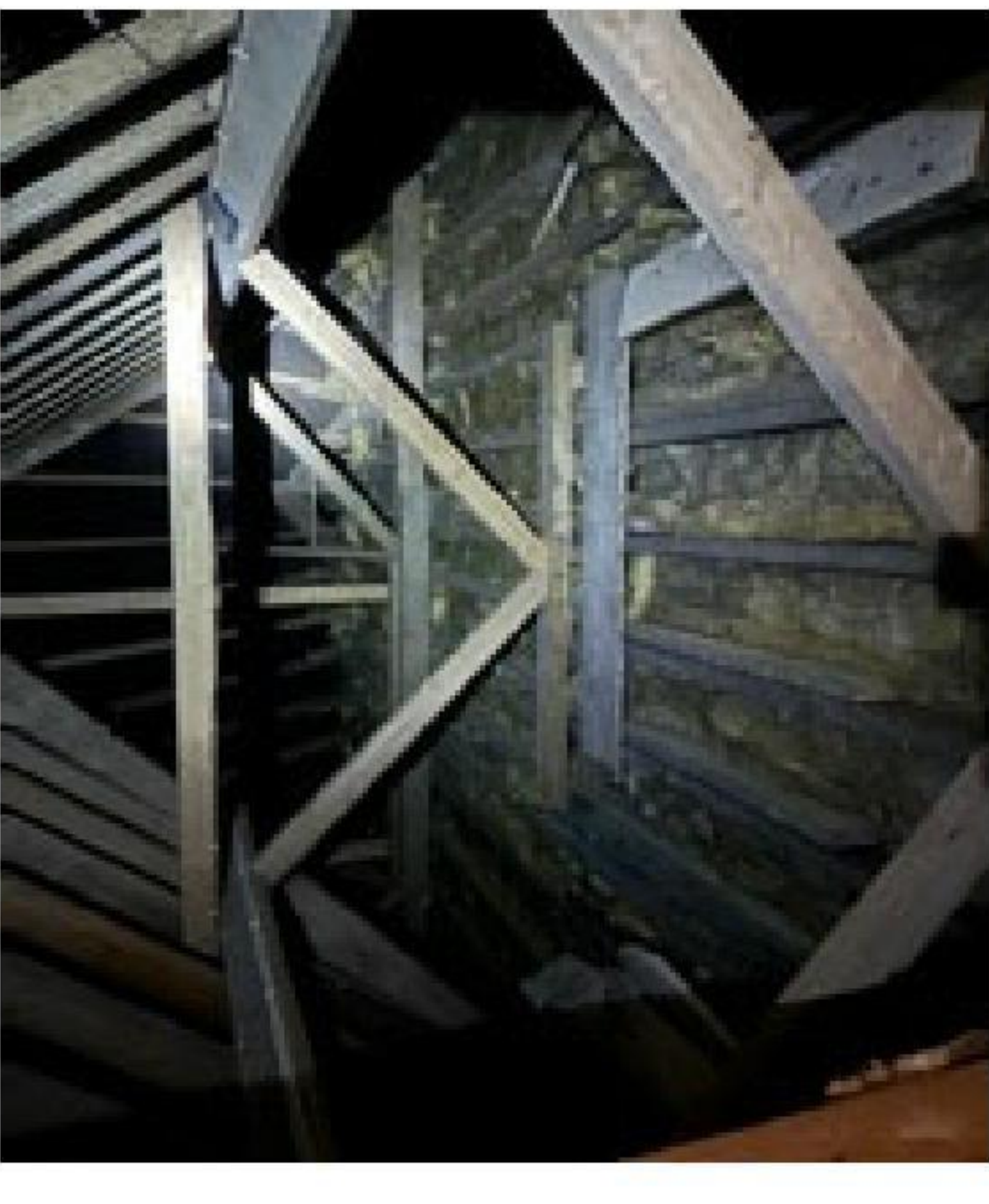
Internal view of roof
