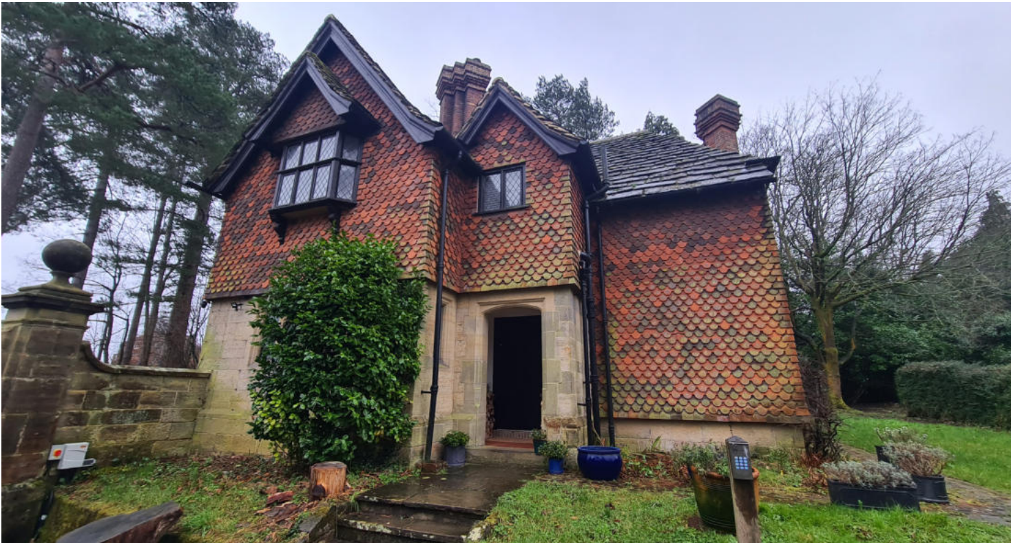
North side of South Lodge
