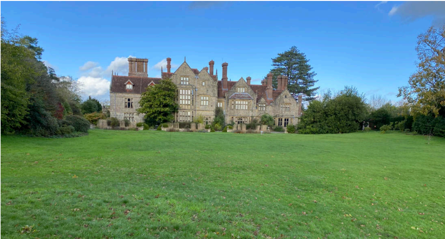
South Front of Borde Hill Place
