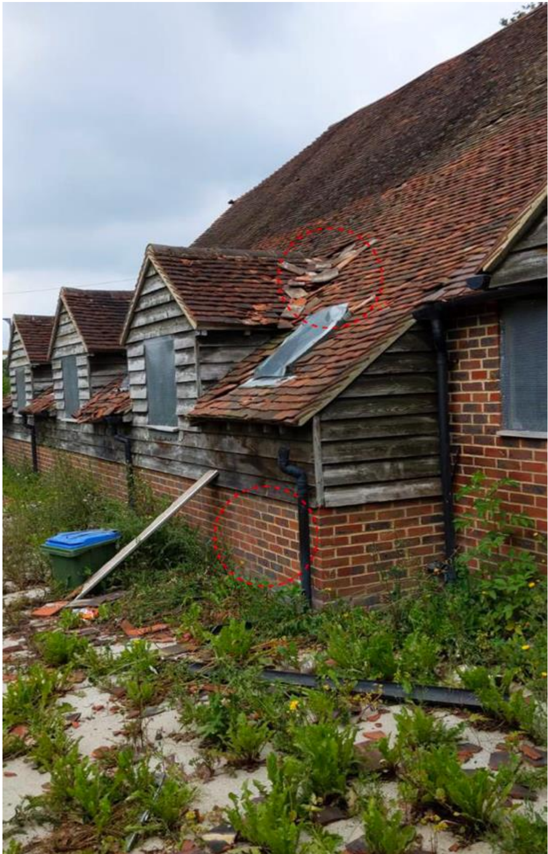
Southern elevation illustrating alterations
