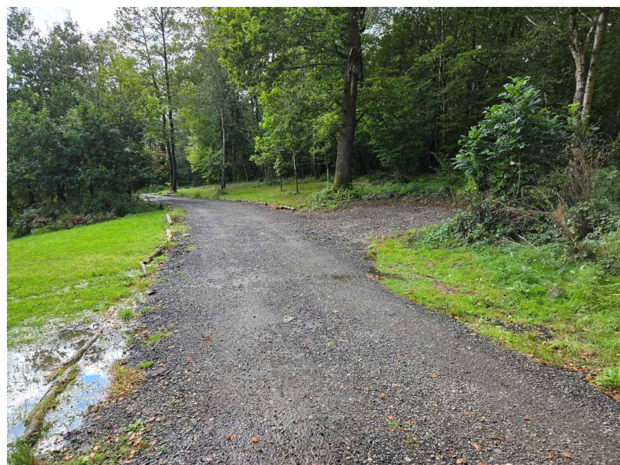
View 7. Existing track from south pod.
