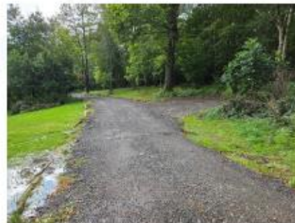
View 7. Existing track from south pod.
