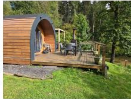
View 1. Facing east overlooking south pod and decking .
