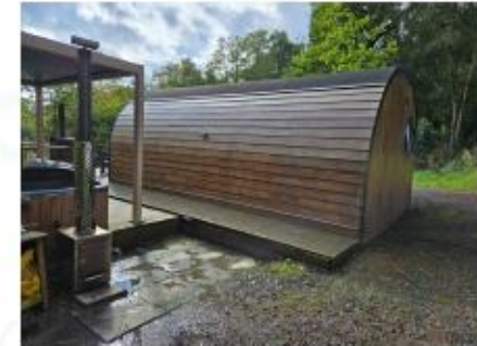
View 3. Rear view of the south pod and deck.
