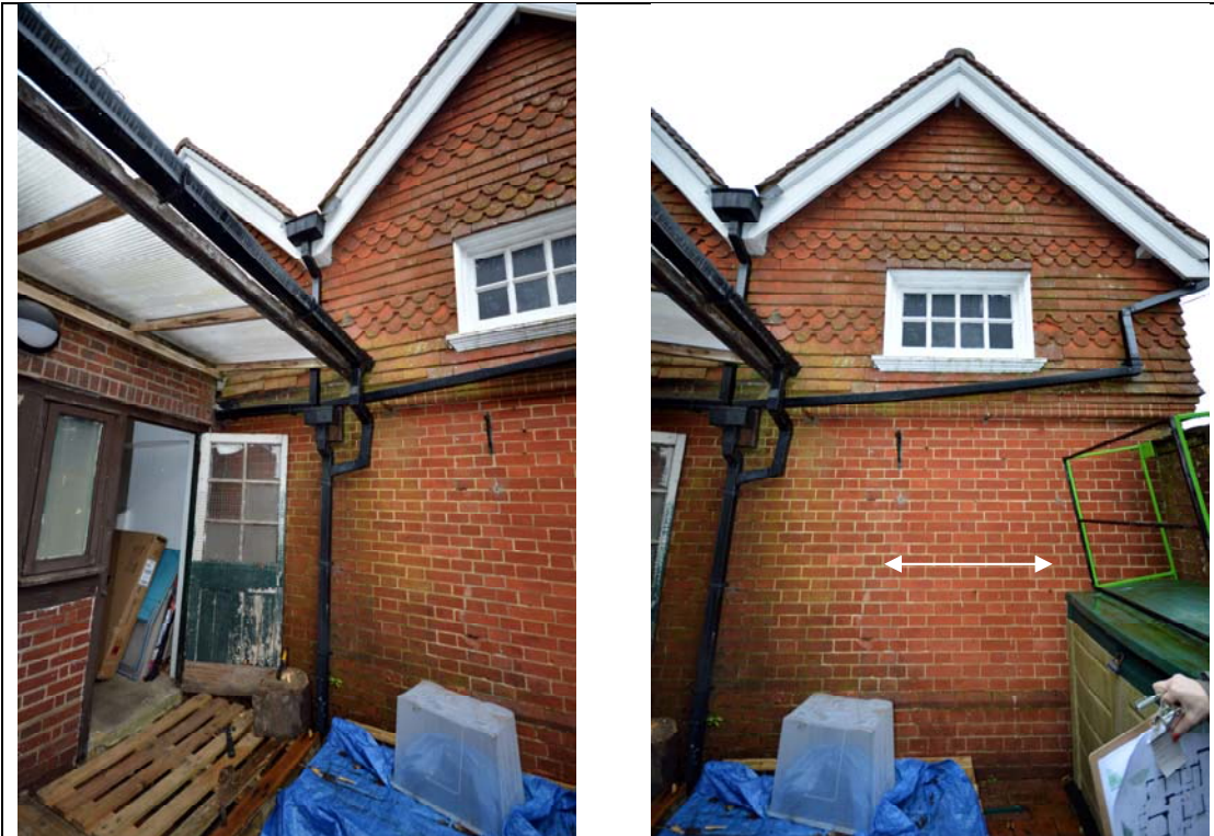
Plate 28: The south elevation of the former stable block and the suggested location for the new opening (arrow)
