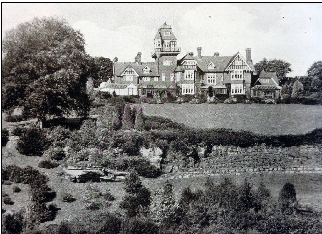
Plate 6: The garden front from the east side in 1926 showing the topography of the site and the extent of architectural embellishments (West Sussex Record Office reference: SP 645)
