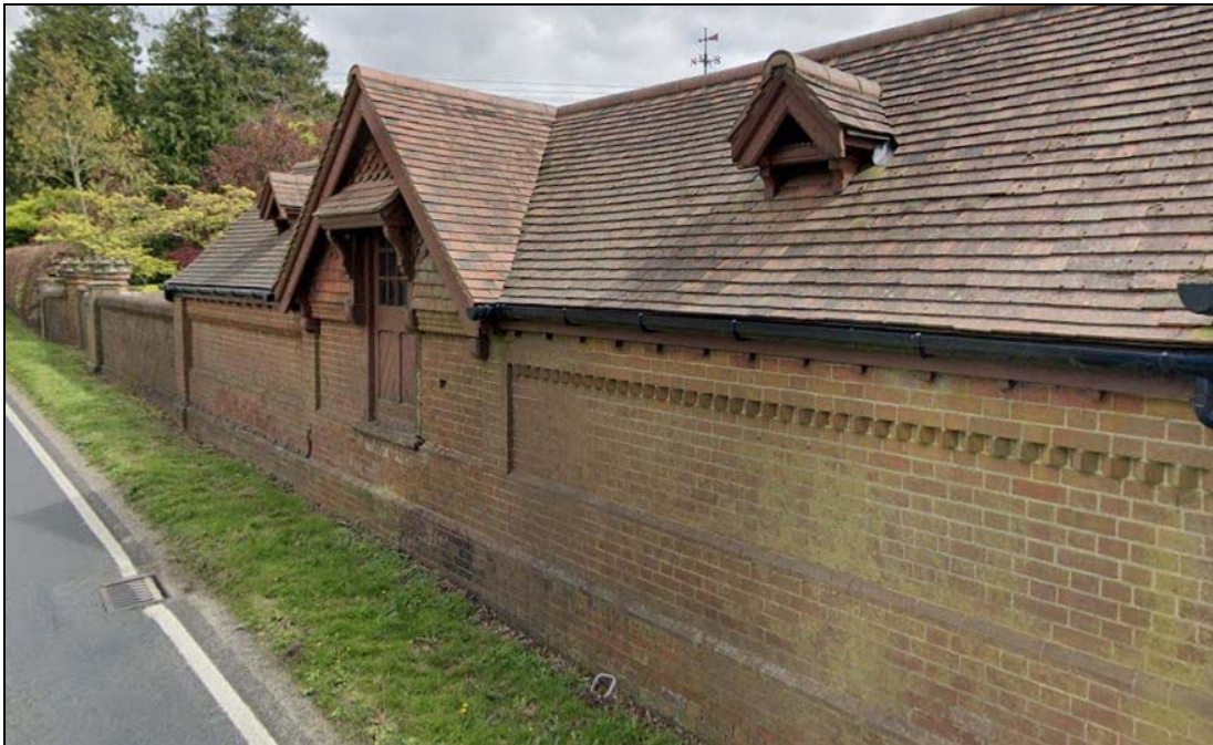
Plate 24: The north end of the group on the west side showing the second loading doorway and the pair of roof vents
