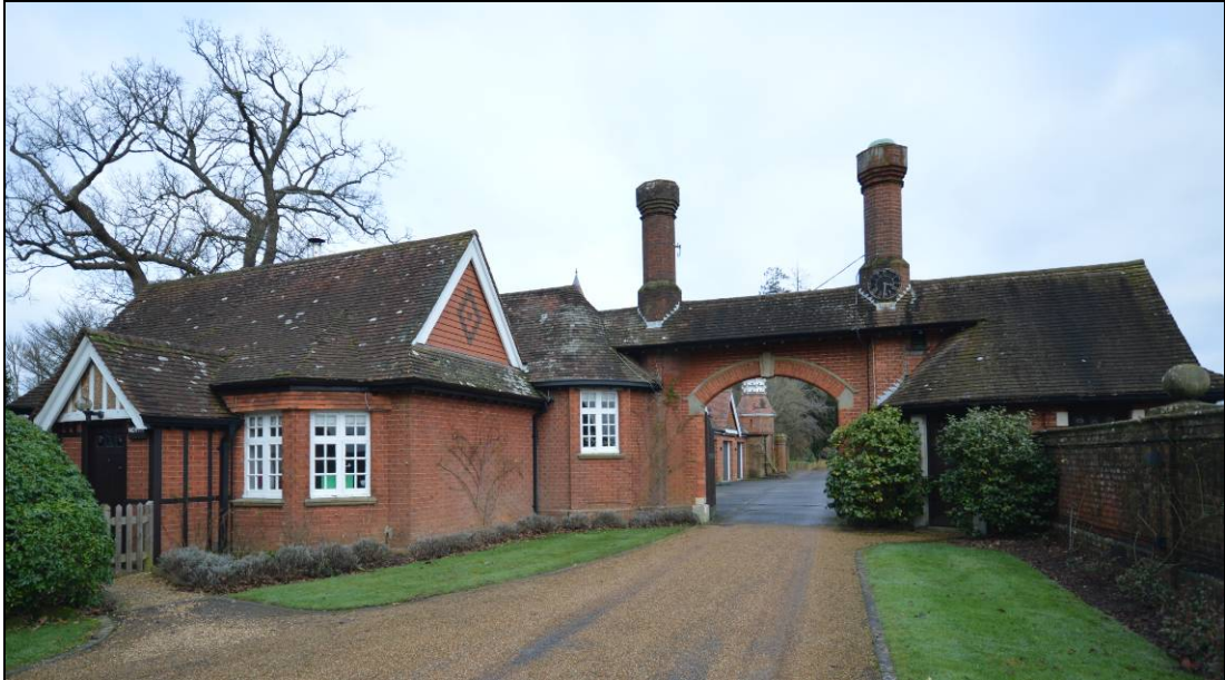
Plate 14: The south side of the domestic part of the group with the arched entrance-way between the two separate parts of the North Lodge showing the quality and consistency of the brickwork
