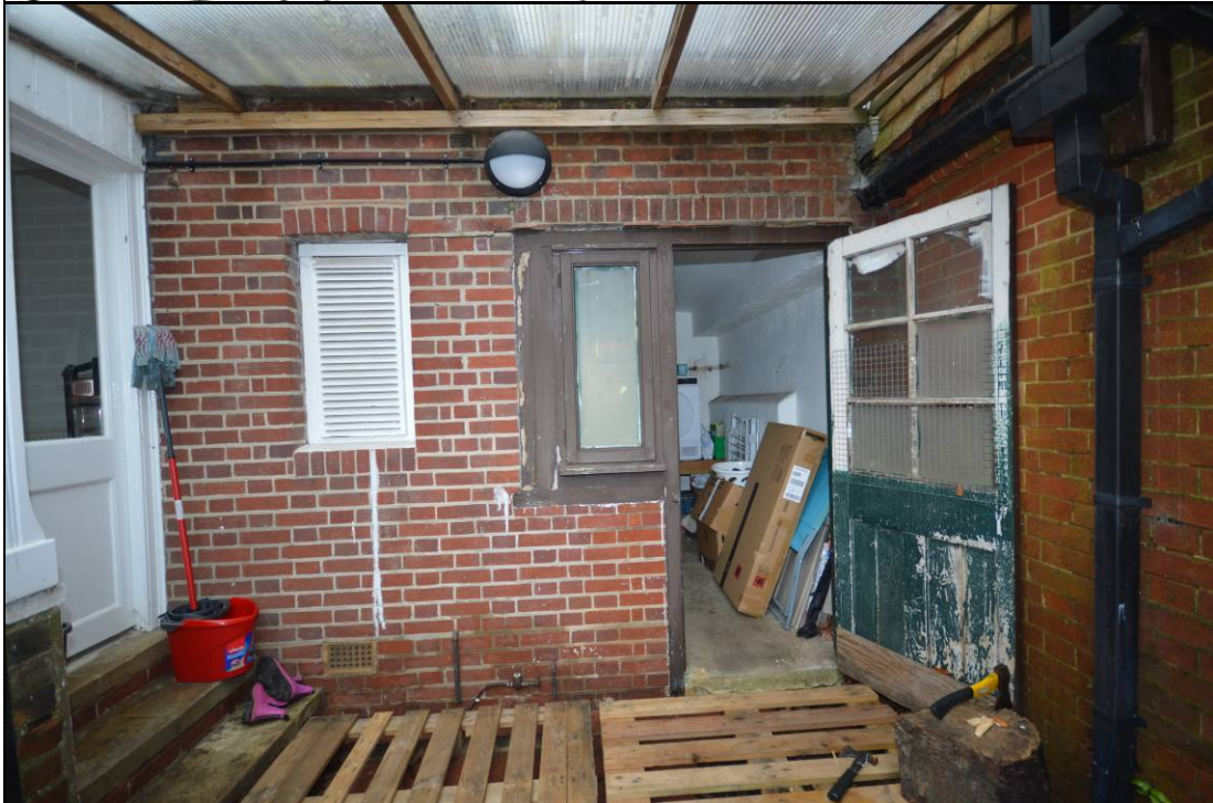
Plate 13: The west elevation of the covered part of the east yard showing the Flemish bond brickwork and the integral openings (glazing renewed at a later date)
