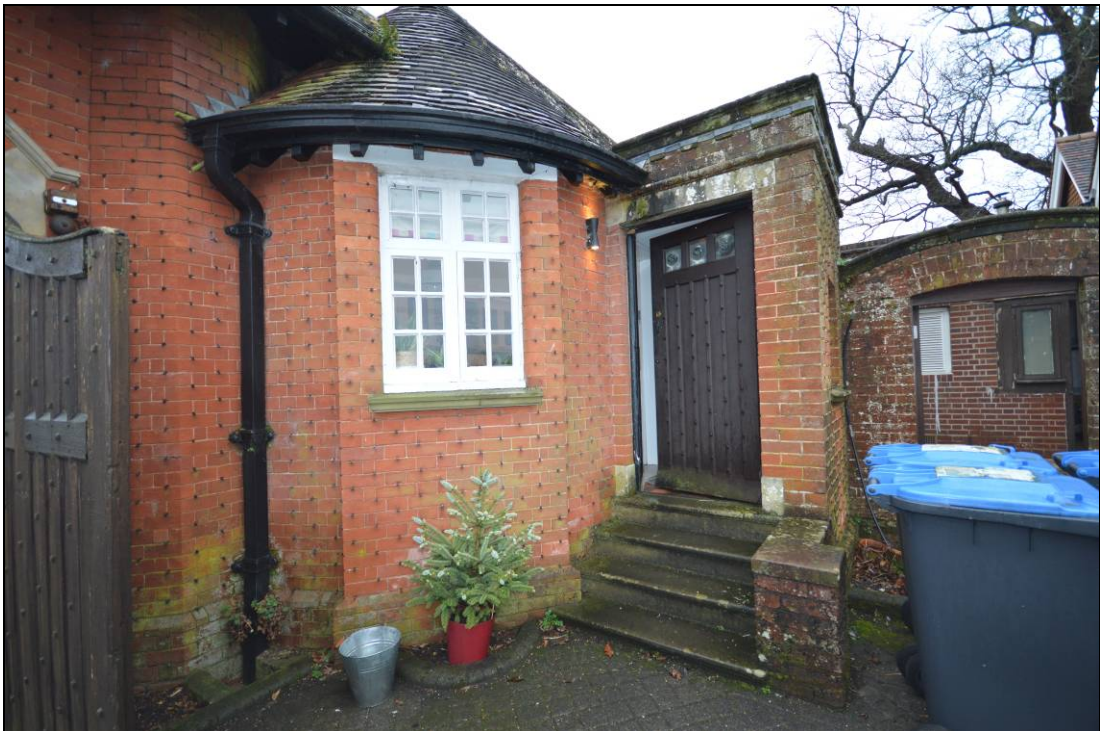
Plate 15: The rounded north side of the Kitchen and the porch showing the quality of the brickwork
