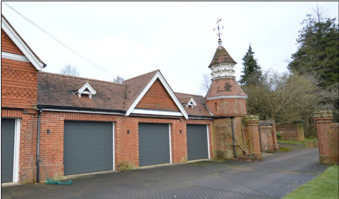
Plate 22: The east elevation of the northern part of the stable and garage block group
