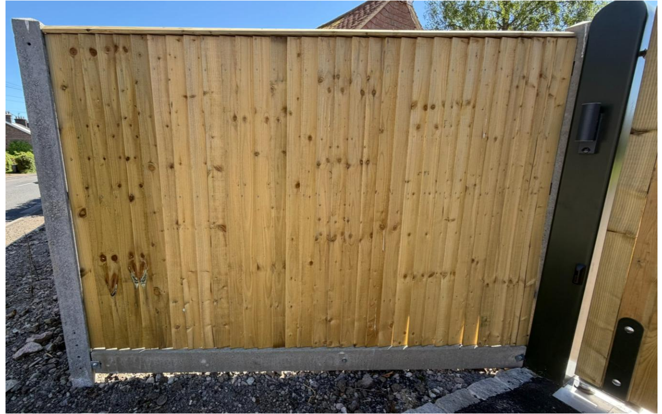
1800 mm high natural wood closed-board Fence with concrete posts and gravel boards
