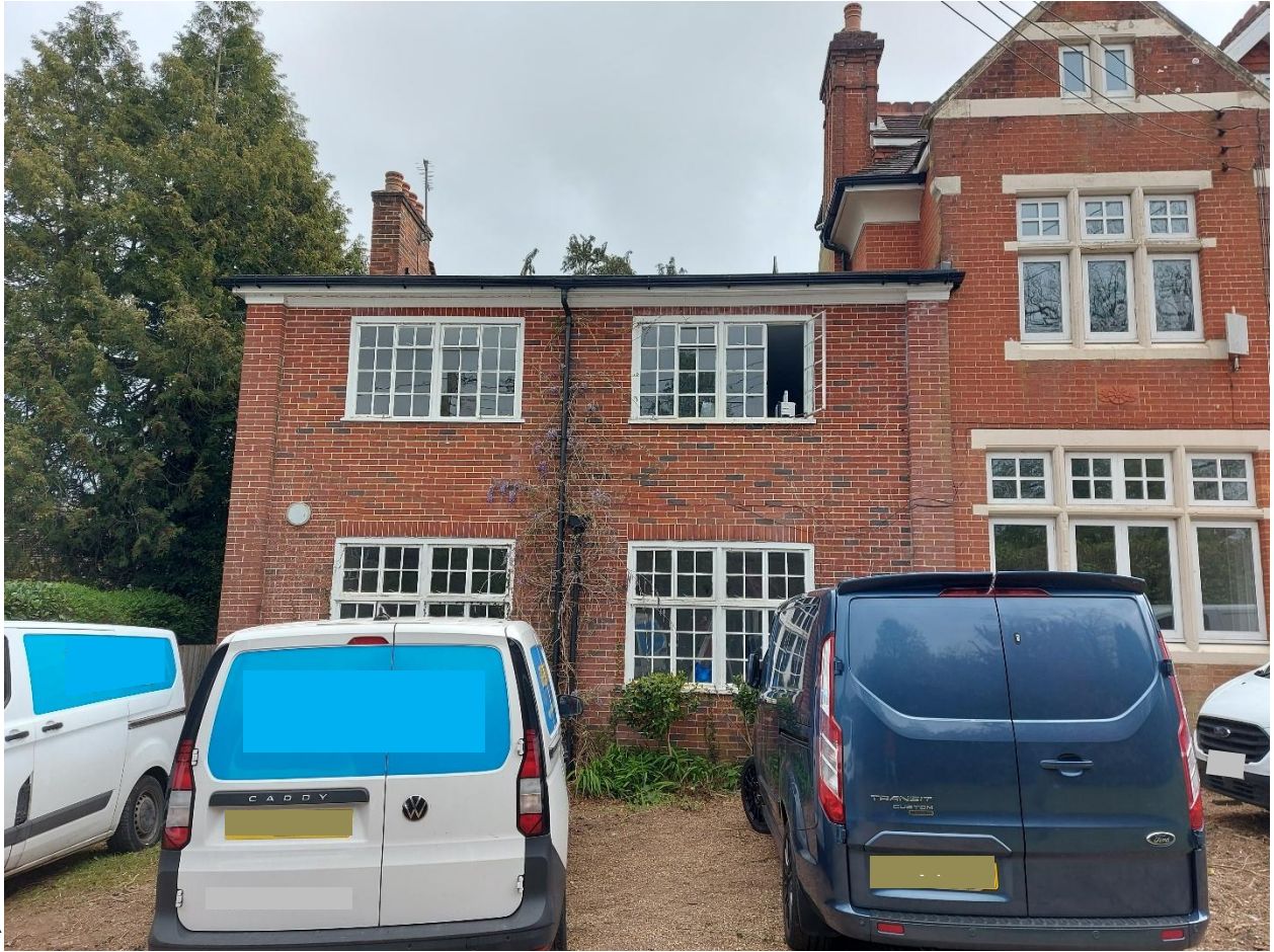
West elevation of the existing extension
