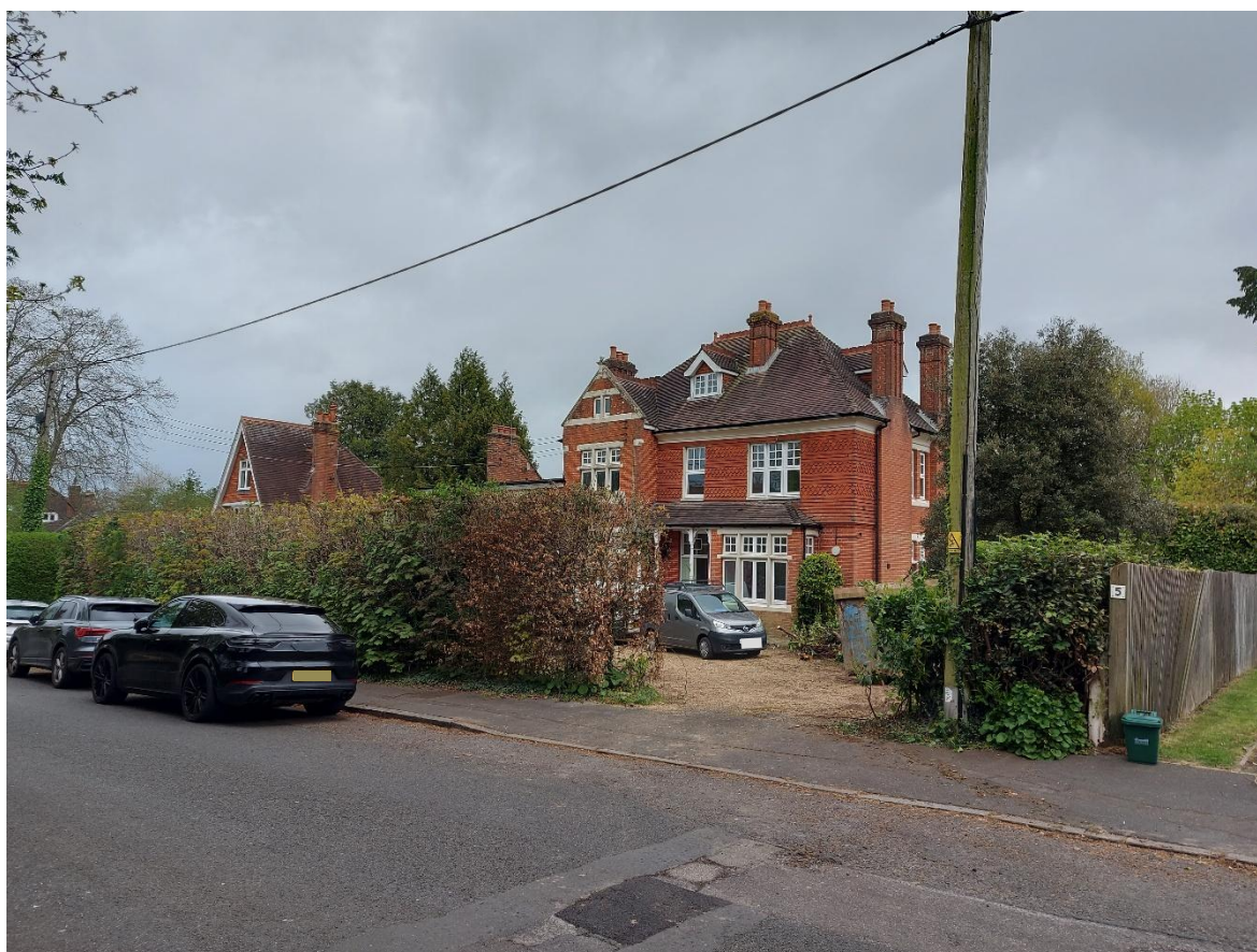
Existing South Entrance
