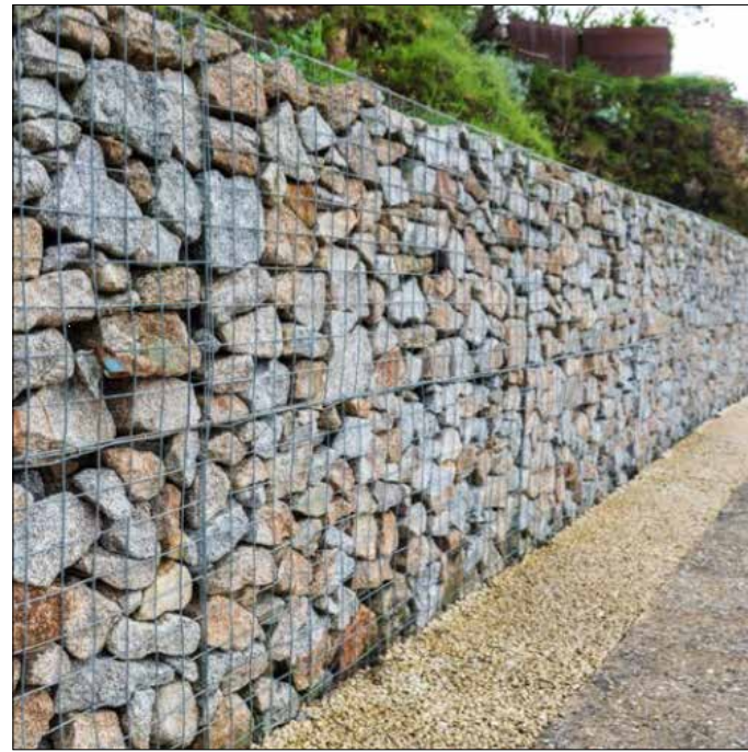
Retaining Features: Gabion Baskets.
