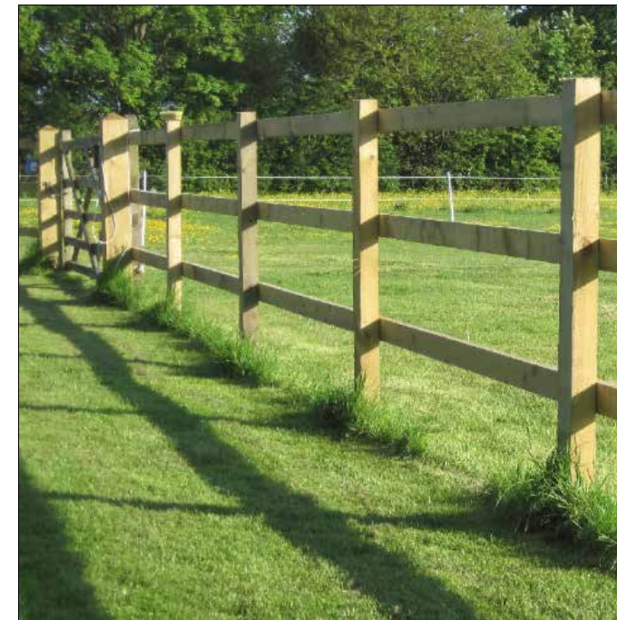
Edge Protection: Timber post and 3-rail fence.
