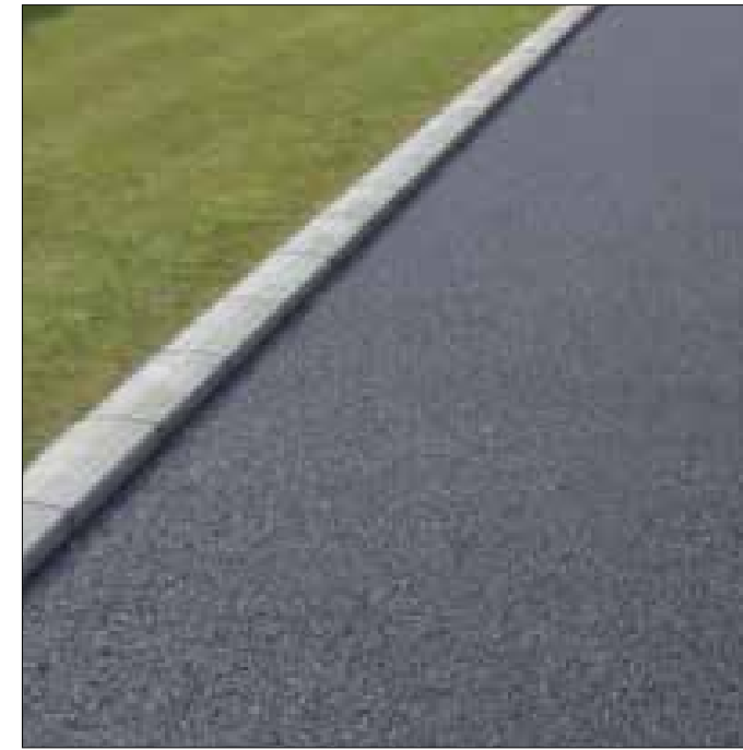
Access roads / paths: Tarmacadam surface.
