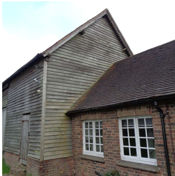
Rear (West Facing) Elevation
