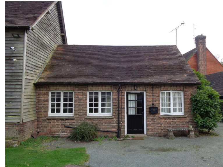
Rear (West Facing) Elevation
