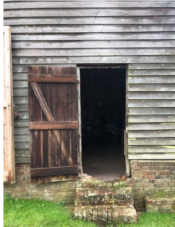
Repair and make good any existing feather-edge timber cladding.
