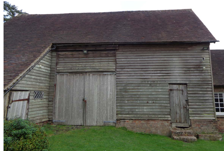
Rear (West Facing) Elevation
