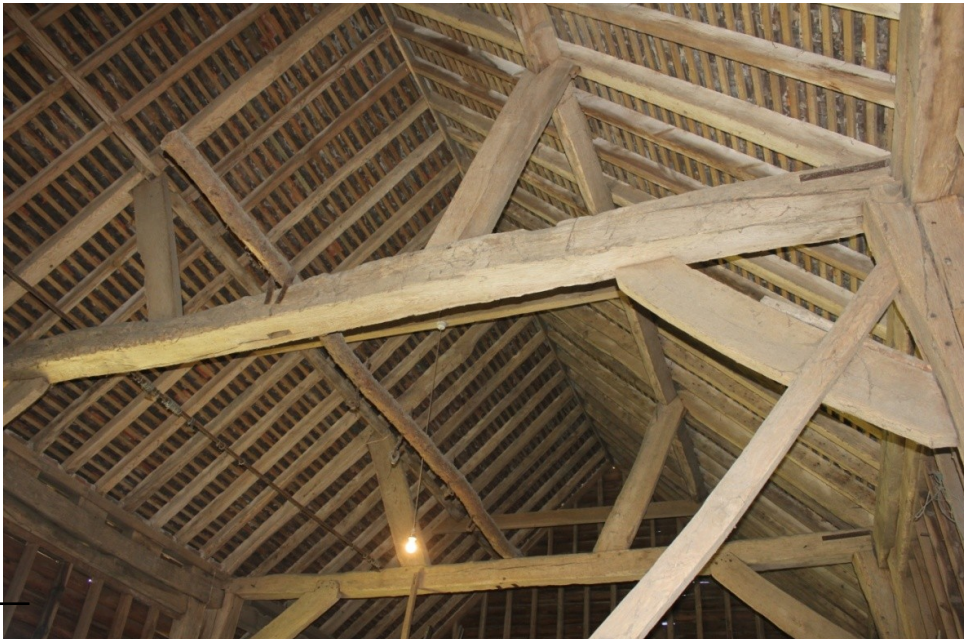
All roof timbers and structure to remain in tact.
