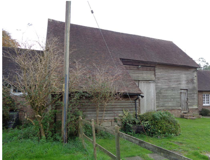
Rear (West Facing) Elevation
