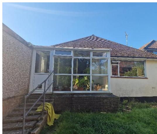
Rear Elevation (showing conservatory and garage to left – both to be demolished)
