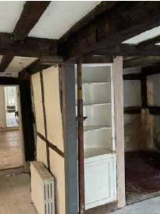
Pre-construction photograph - steel post supporting timber frame
