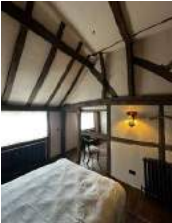
View from north bedroom towards altered wall (timber frame remaining)
