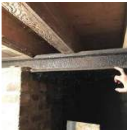
Pre-construction basement, railway steel member used for structural support, now replaced as per Structural Engineer proposal
