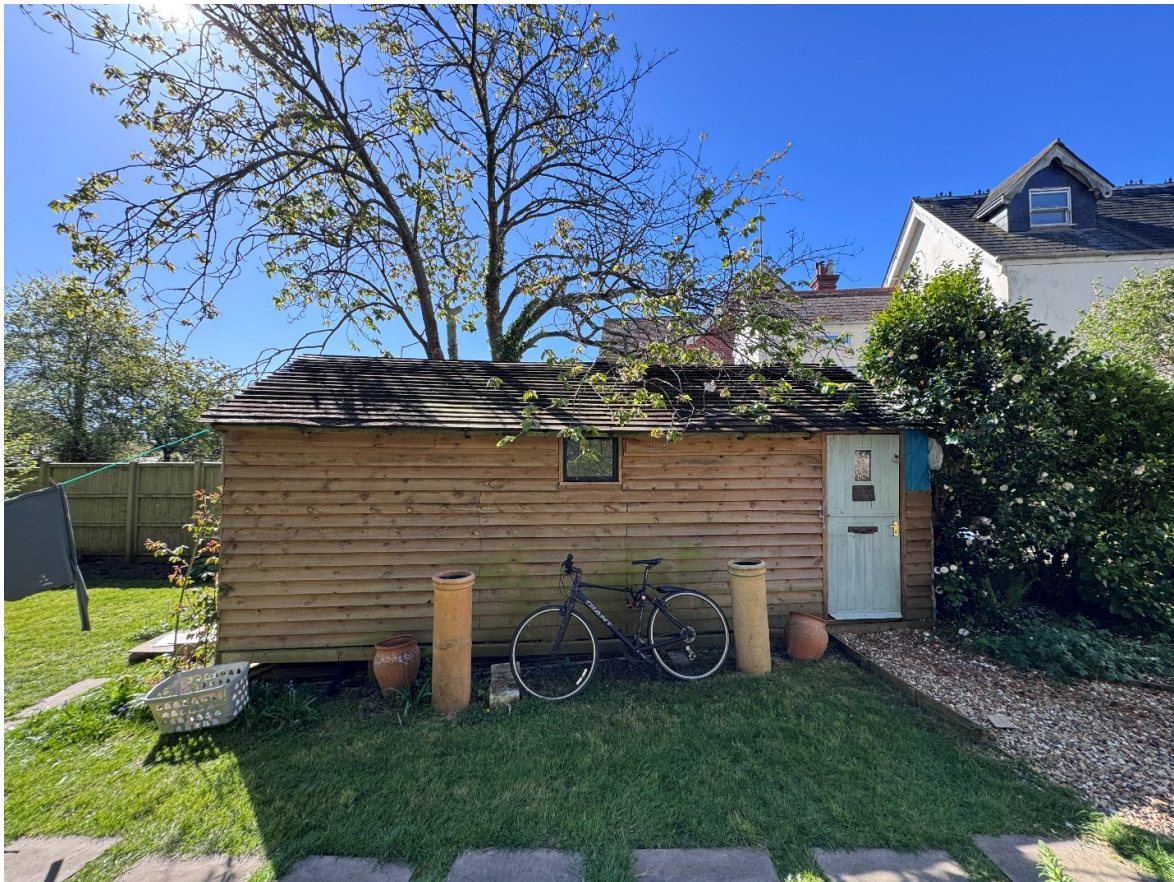
Fig.1 – Existing Garden Shed
