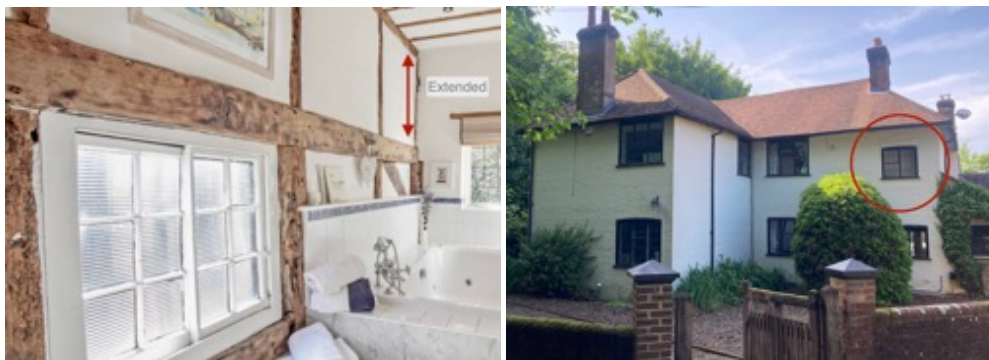
The extended timber-frame in the bathroom and window set low, well below the eaves.
