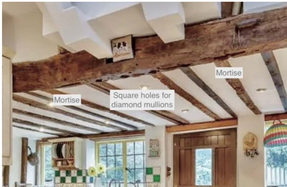
The beam in the kitchen containing evidence of a former window.
