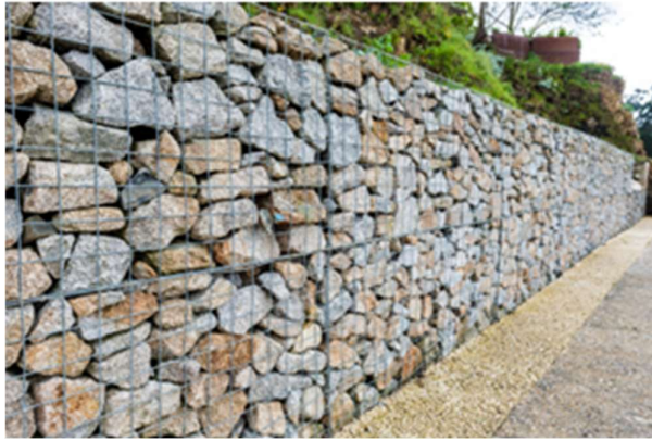
Figure 13 – Modern basket retaining wall
