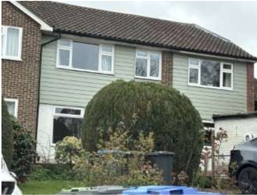
Figure 22 – Trinity Road, Hurstpierpoint (significant cladding)
