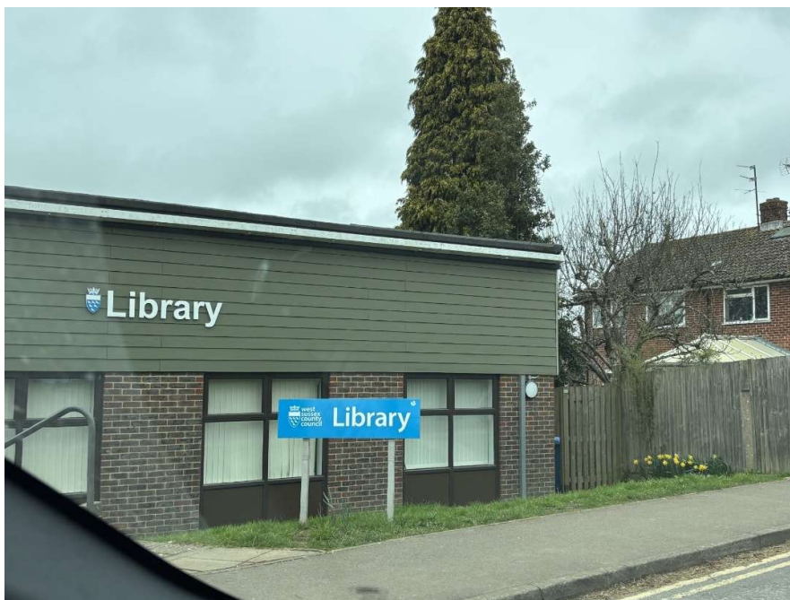
Figure 21 – Trinity Road, Hurstpierpoint Library (significant cladding)
