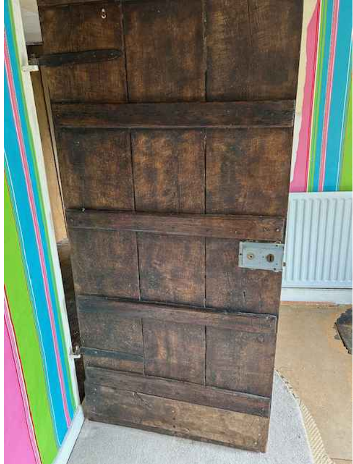
Existing timber door to be re-instated and fixed shut
