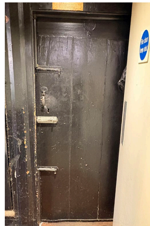
View of cellar door from outside the cellar
