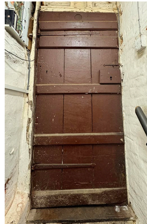
View of cellar door from inside cellar - the direction in which it will be pinned back
