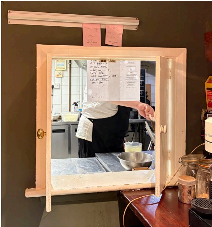
View of current non-historic serving hatch
