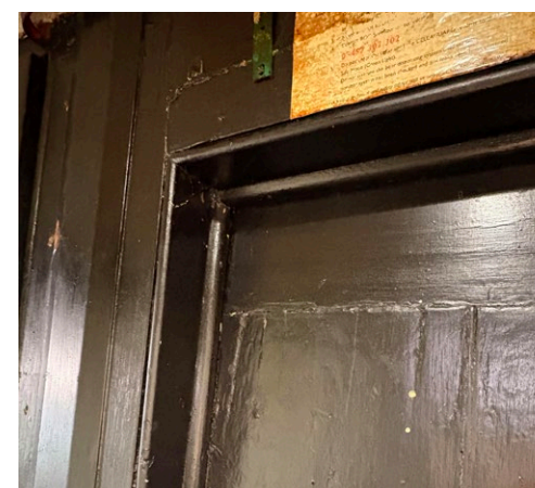
View of cellar door frame from outside the cellar
