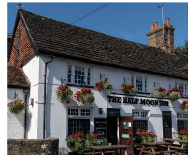
Figure 9: Façade of The Half Moon Inn today
