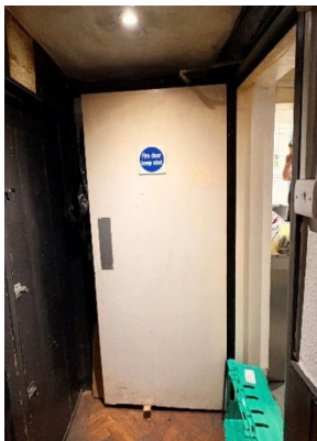
Figure 18: FD1 - One of the non-historic fire doors to be replaced
