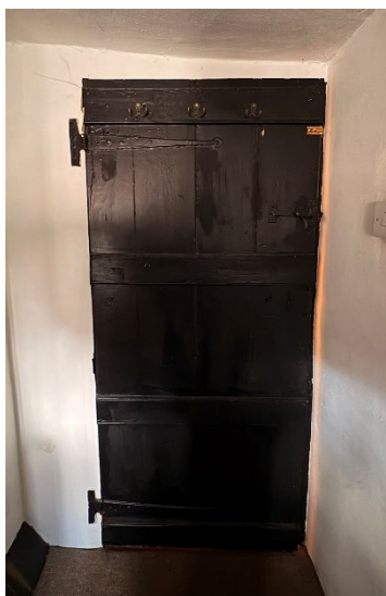
Figure 11: Historic storage room door
