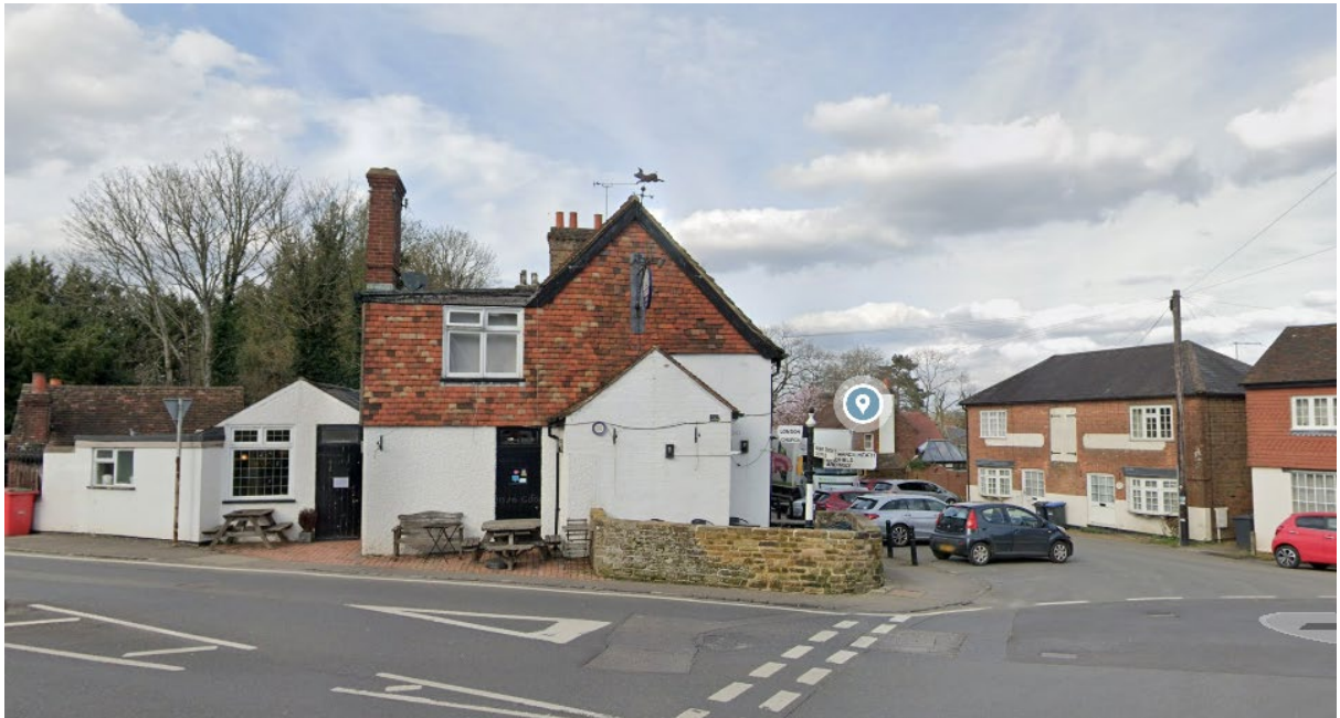
Figure 2: View from South Approach
