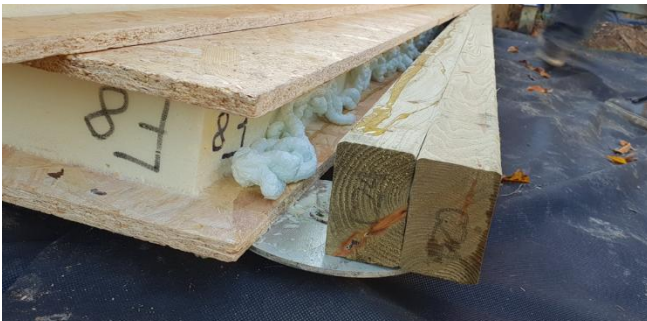
This photo shows how the panels are connected together
