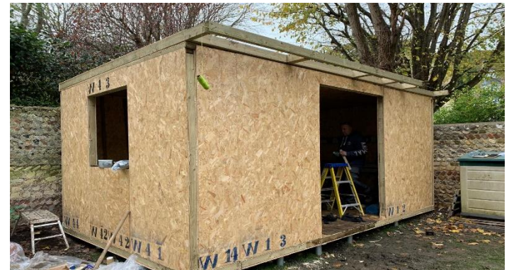
This is how the SIP garden room looks when it is almost finished.
