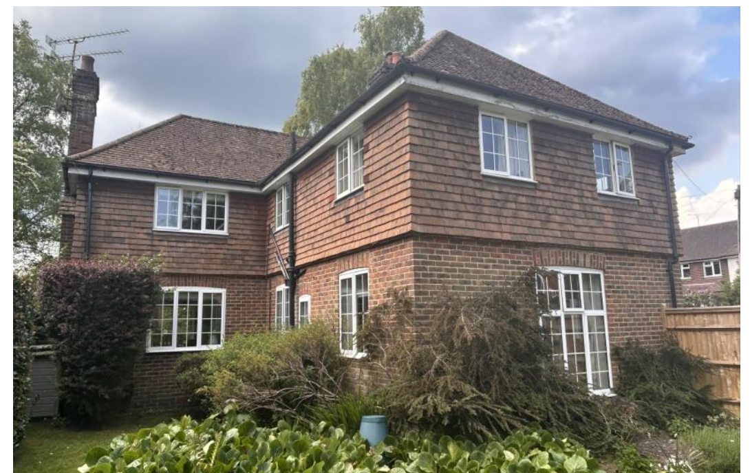
Rear & Side Elevation of The Red House
