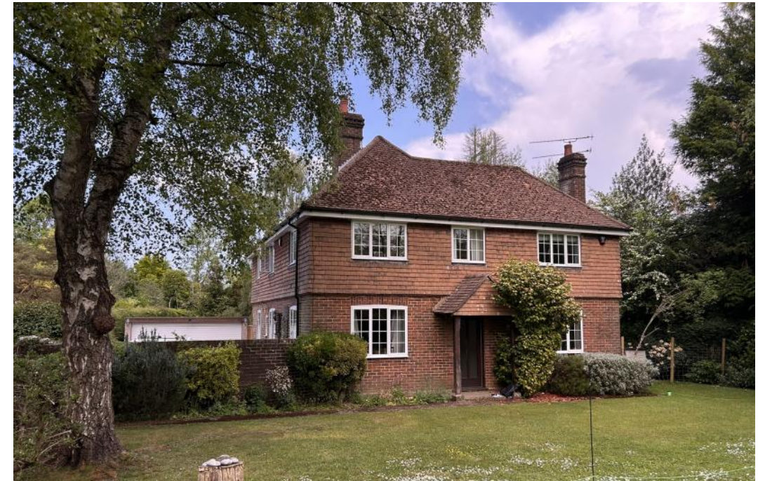
Front Elevation of The Red House facing Lewes Road
