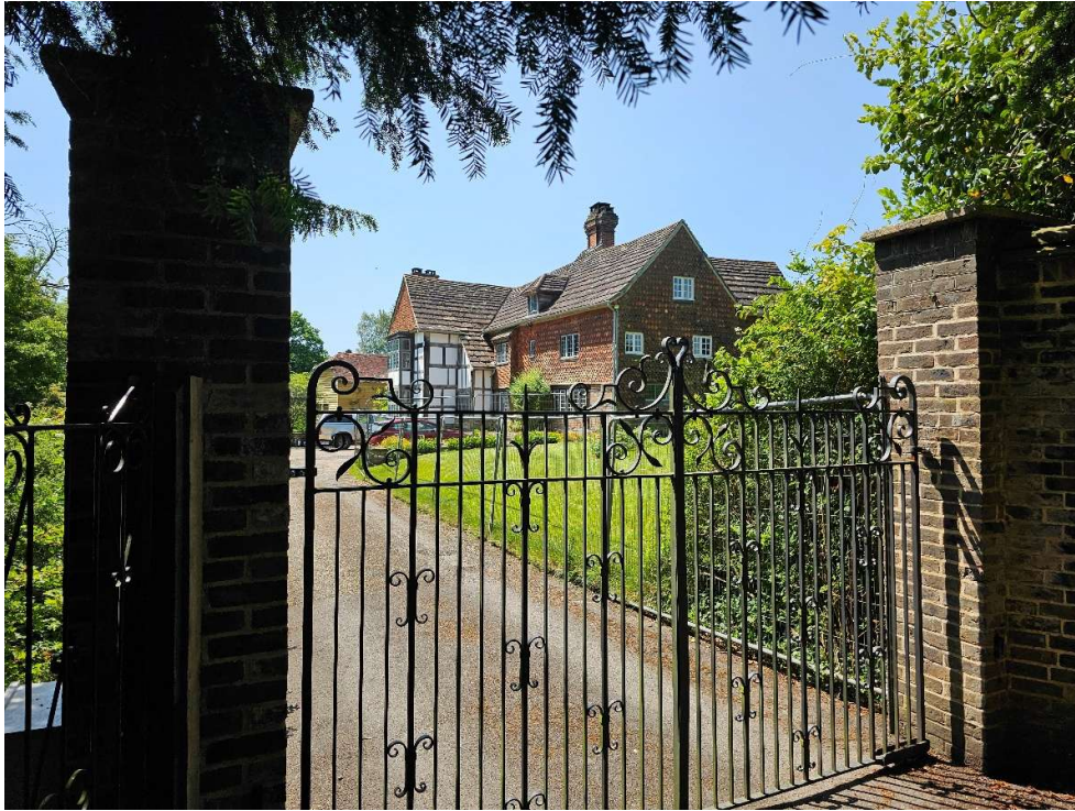
Plate 2: View south from Old Wickham Lane of The Grade II* Wickham Farmhouse.
