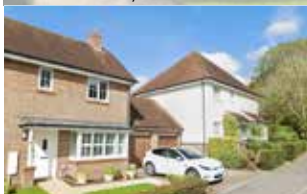
Mix of materials – Renfields
