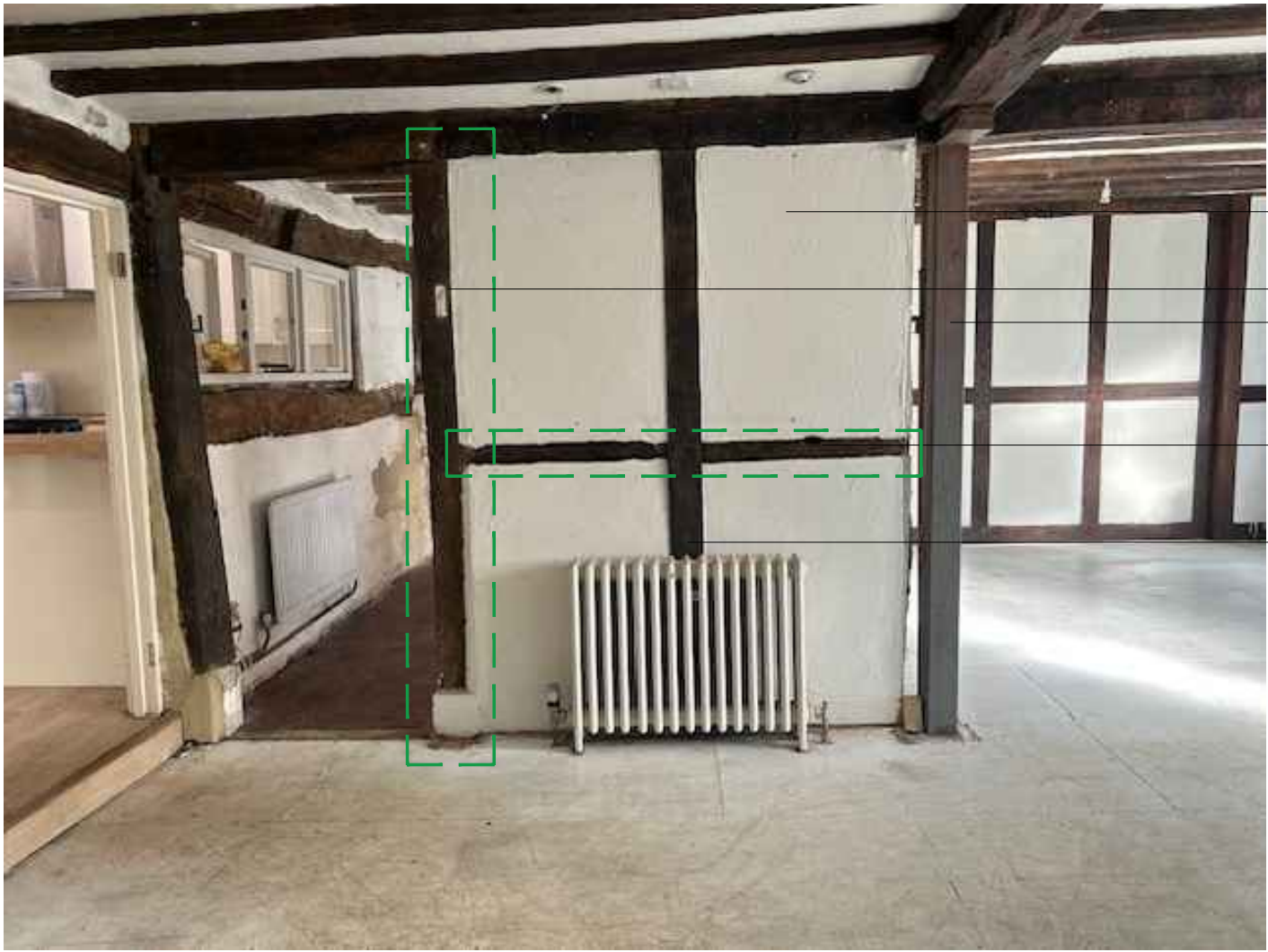
Internal lounge wall prior to changes.
