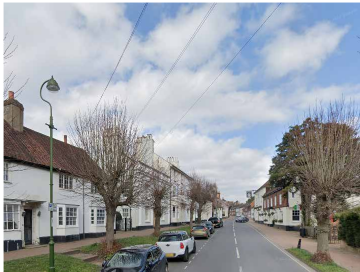
View looking North along High Street
