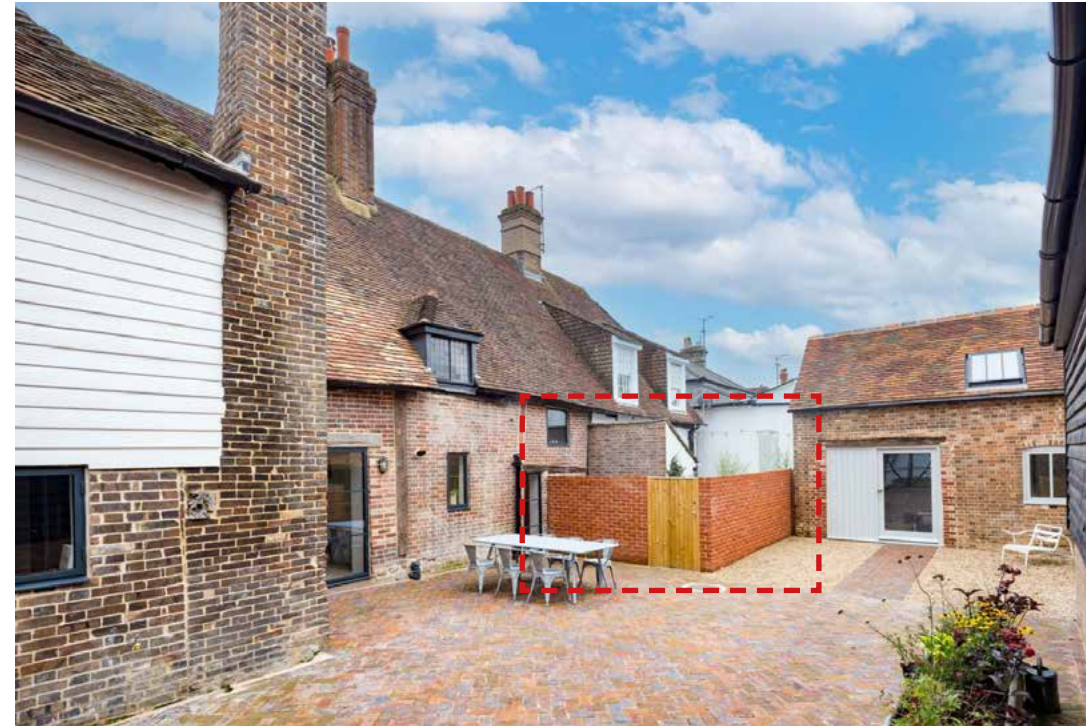
As-built rear brickwork wall
