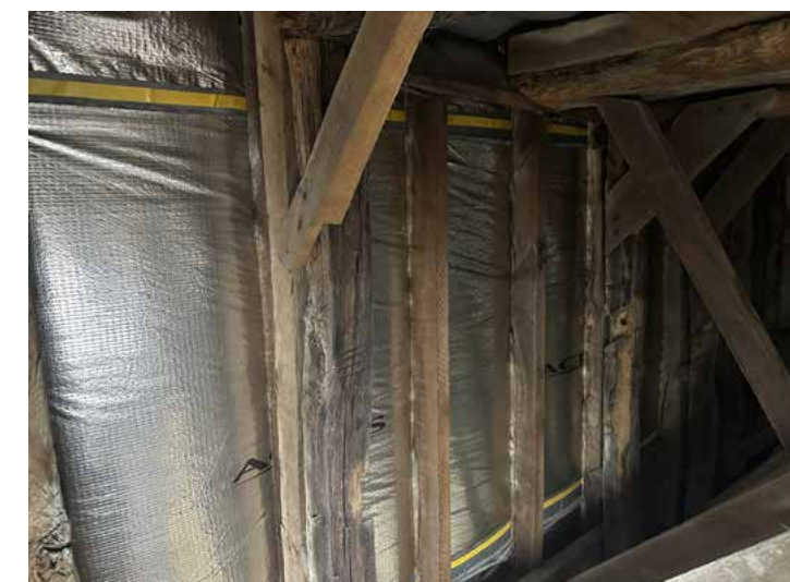
Attic - historic timber frame roof, new insulation
