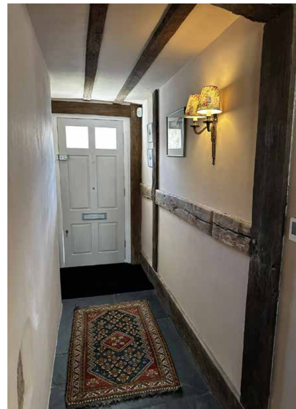
Ground Floor - entrance with old (door jamb and ceiling) and new timber panelling
