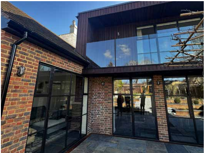
Rear elevation & re-constructed bake house
