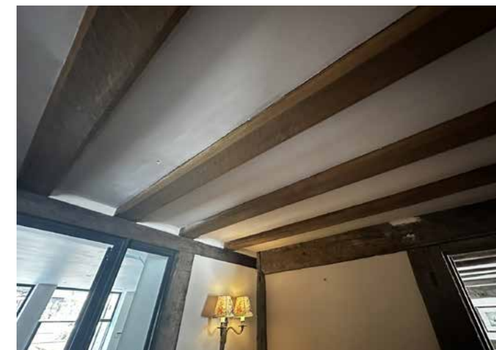
Ground Floor - new timber framing on the Ground Floor ceiling only (infilled void above removed staircase), original timber on walls
