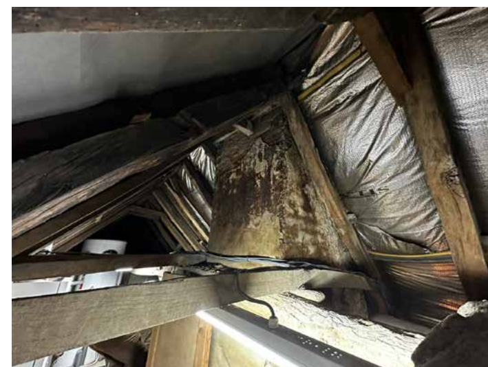
Attic - historic timber frame roof
