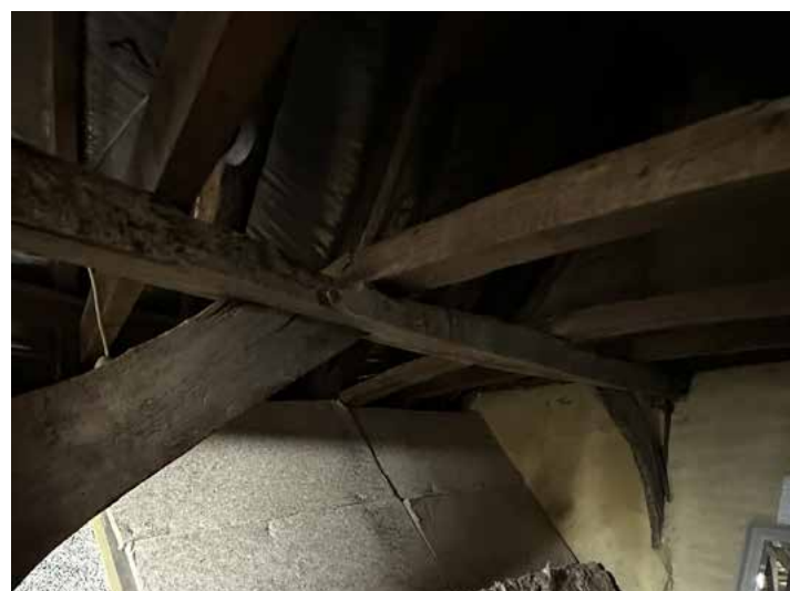
Attic - historic timber frame roof
