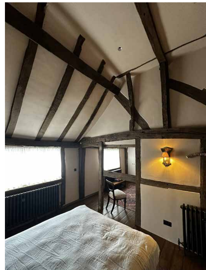
First Floor - historic timber frame roof
