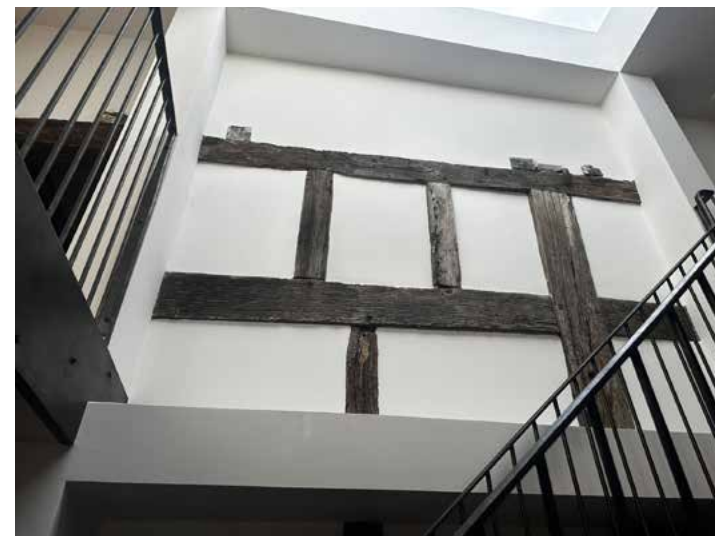
Historic timber frame wall in stairwell
