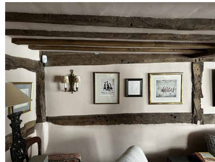
Historic timber frame wall, living room
