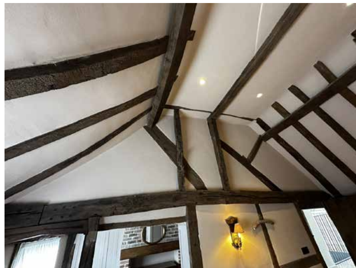
First Floor - historic timber frame roof
