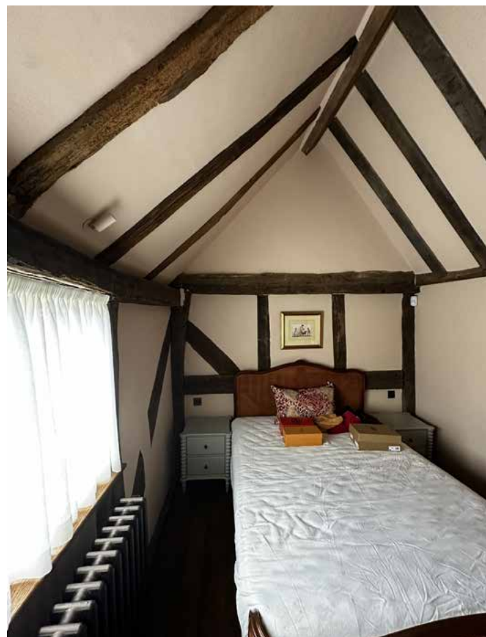
First Floor - historic timber frame roof
