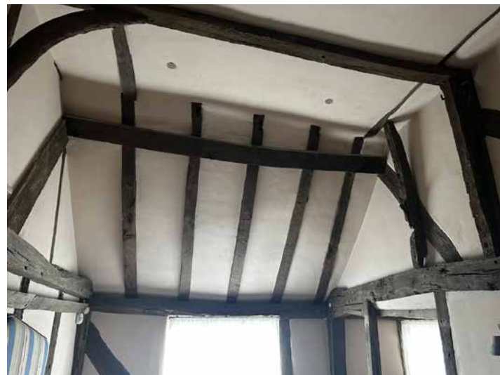
First Floor - historic timber frame roof
