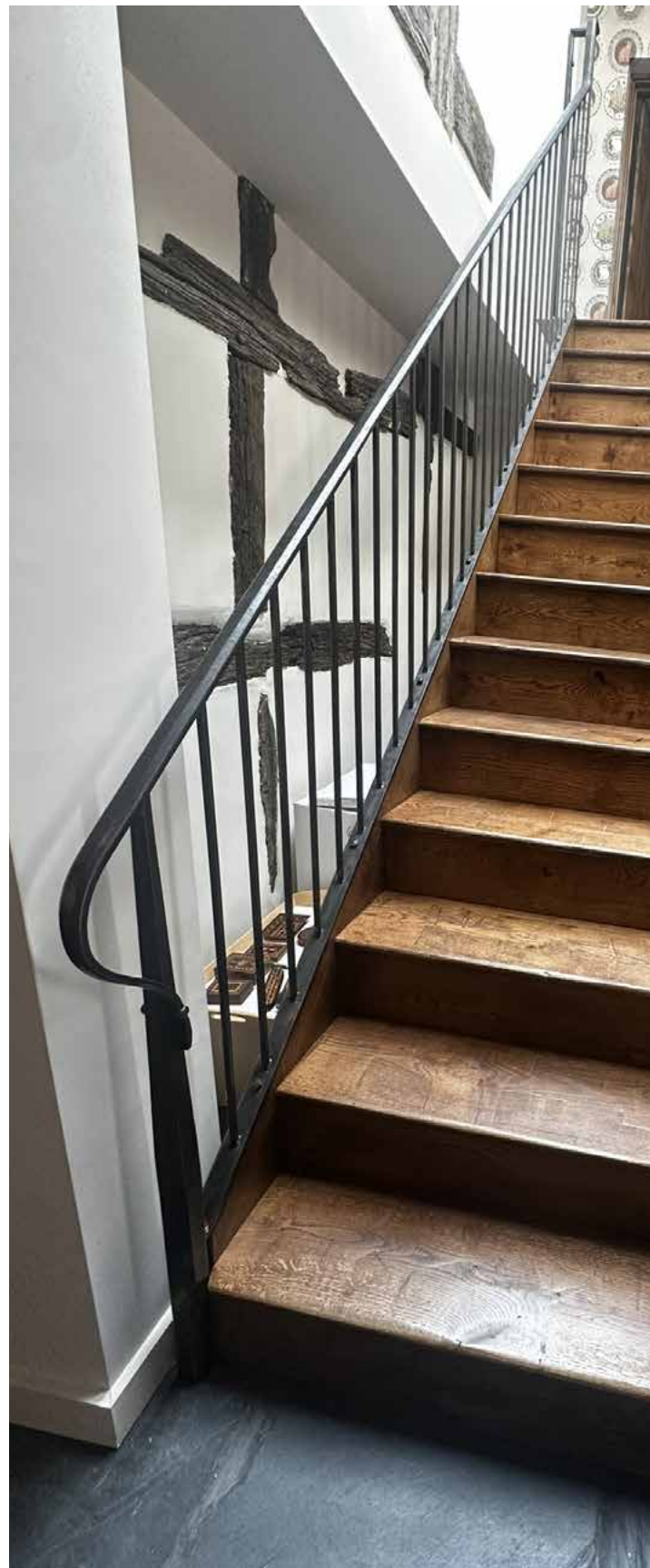
Ground Floor - new staircase in Kitchen/Living/Dining
