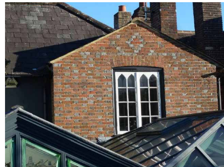
Historic rear extension with gothic window
