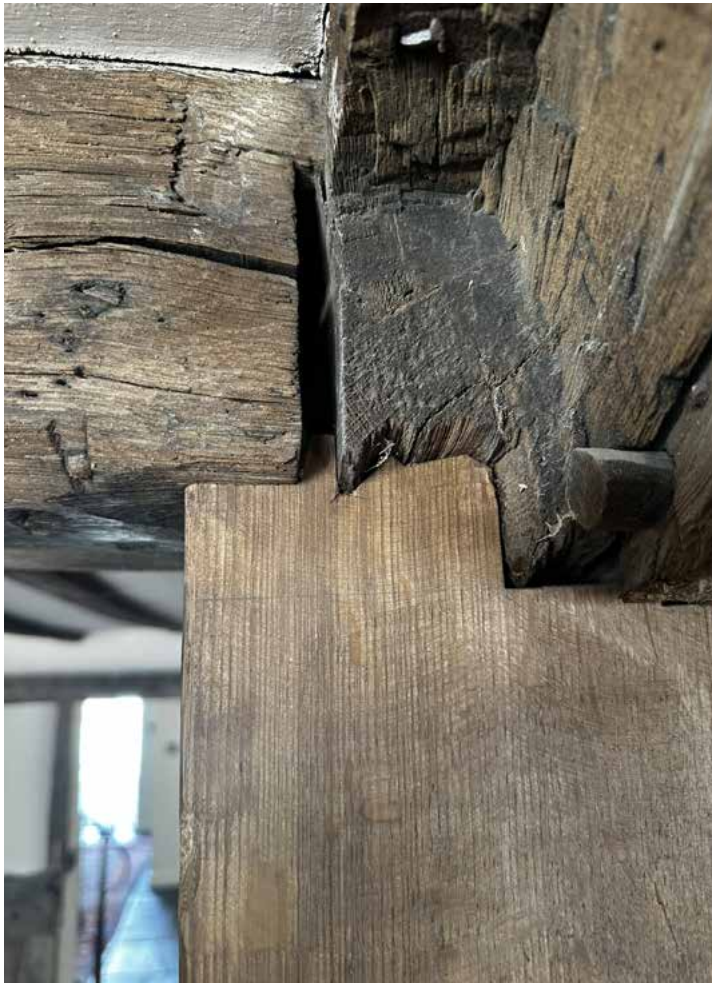
Ground Floor - steel post replaced with timber post
