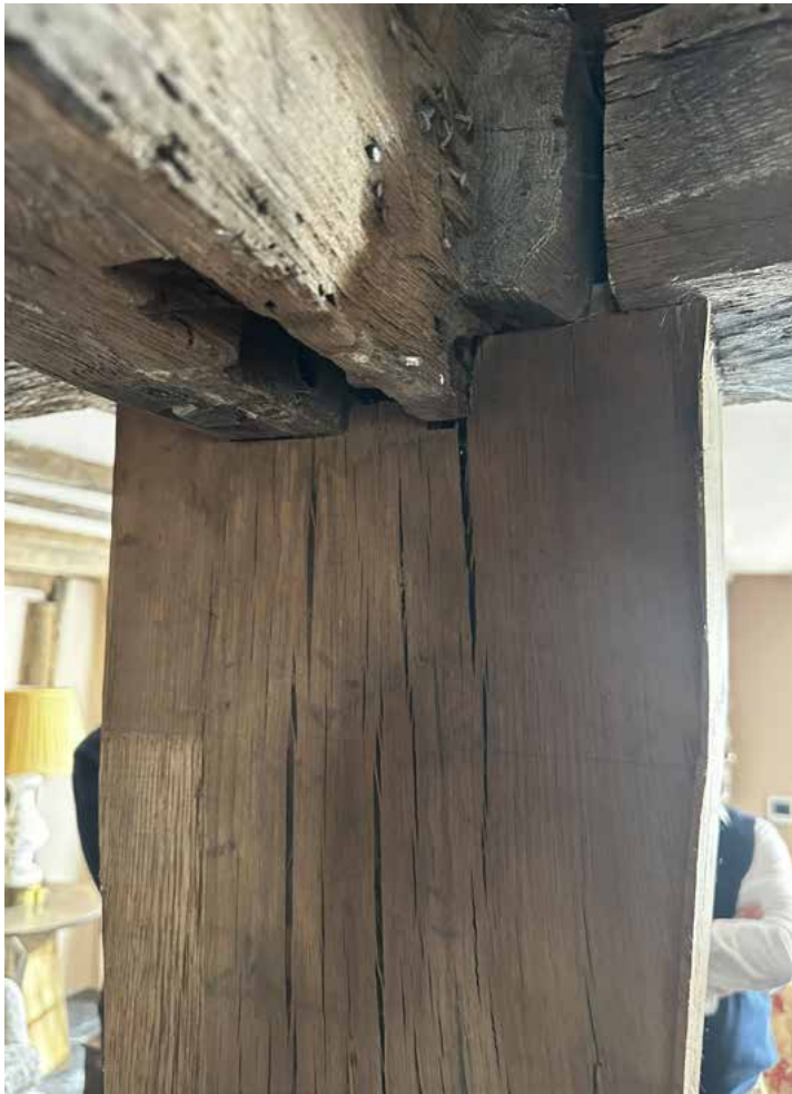
Ground Floor - steel post replaced with timber gunstock post
