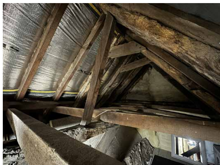
Attic - historic timber frame roof
