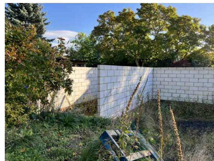
Garage walls constructed
