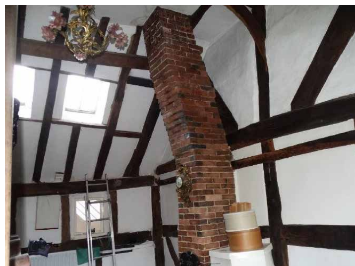
First floor bedroom, chimney stack
