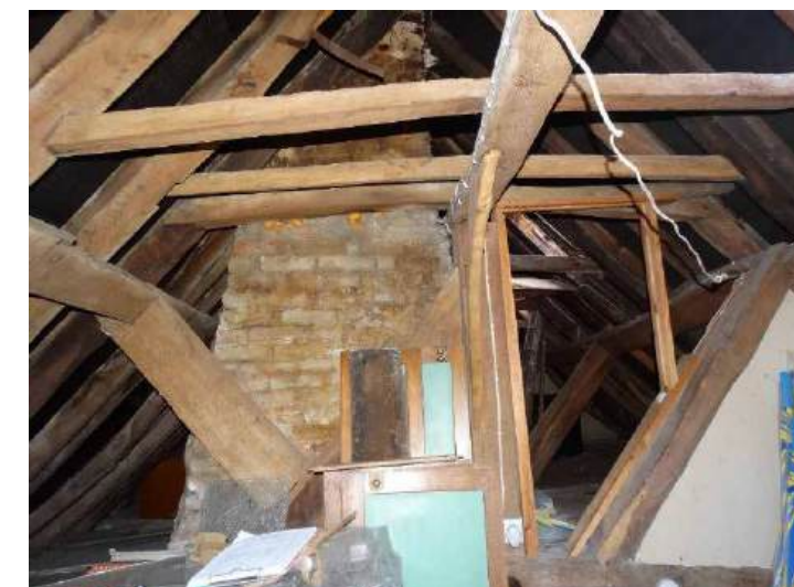
Attic, chimney stack in the background
