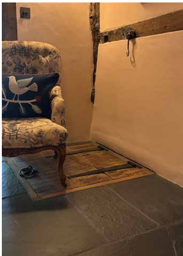
Ground Floor -access hatch to basement
