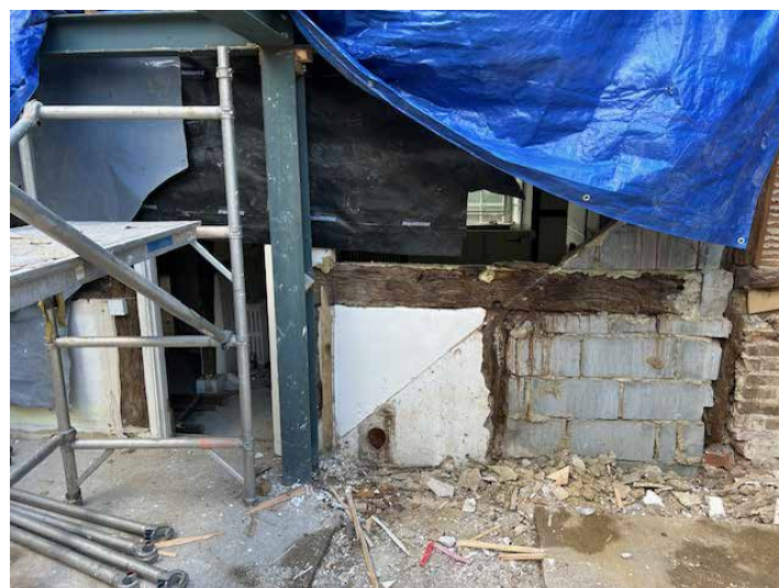
Breeze block within external and internal walls
