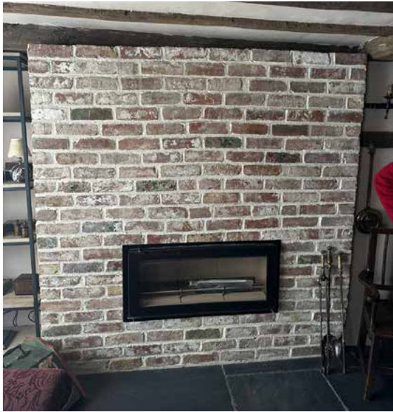
Ground floor living room re-faced chimney breast
