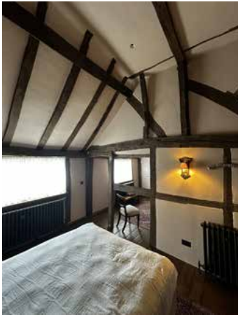
View from north bedroom towards altered wall (timber frame remaining)
