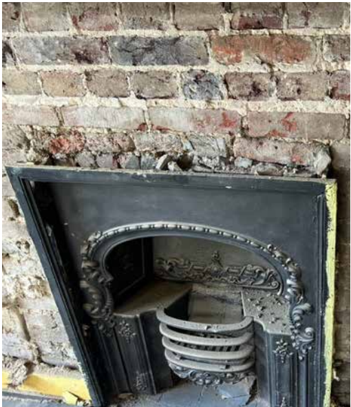
First floor bedroom fireplace and chimney breast before works
