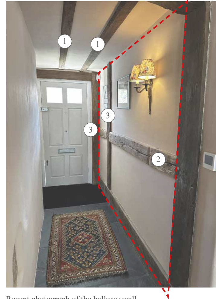
Recent photograph of the hallway wall
