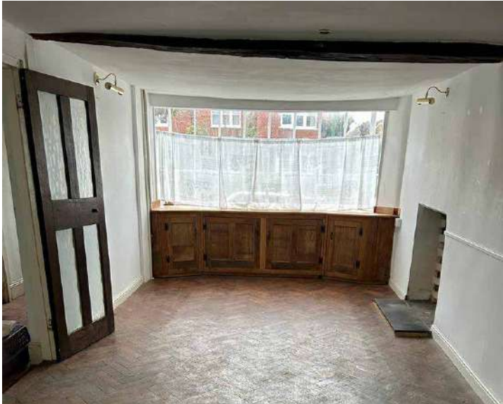
Ground floor study fireplace before works- opening on the right side
