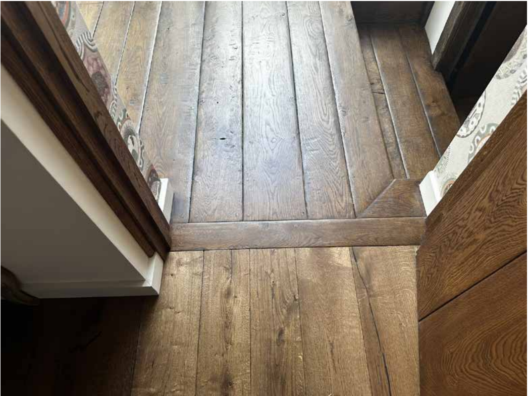
As-built oak flooring
