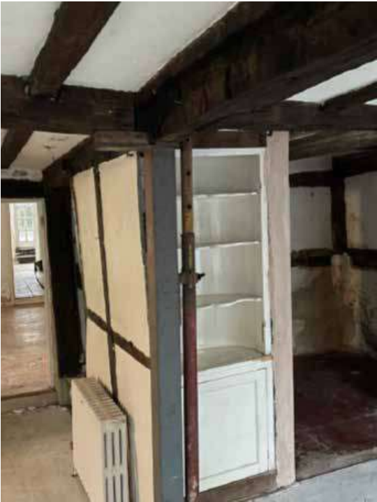
Pre-construction photograph - steel post supporting timber frame
