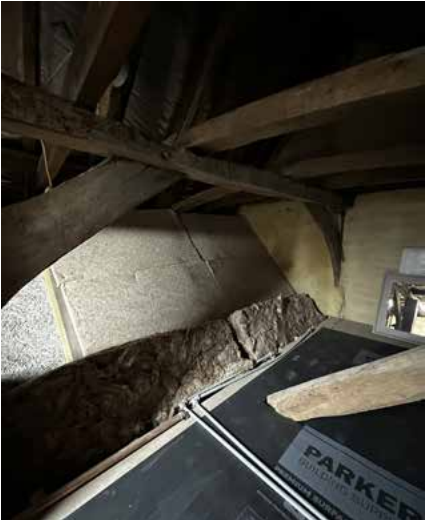
Attic, view of the vaulted ceiling
