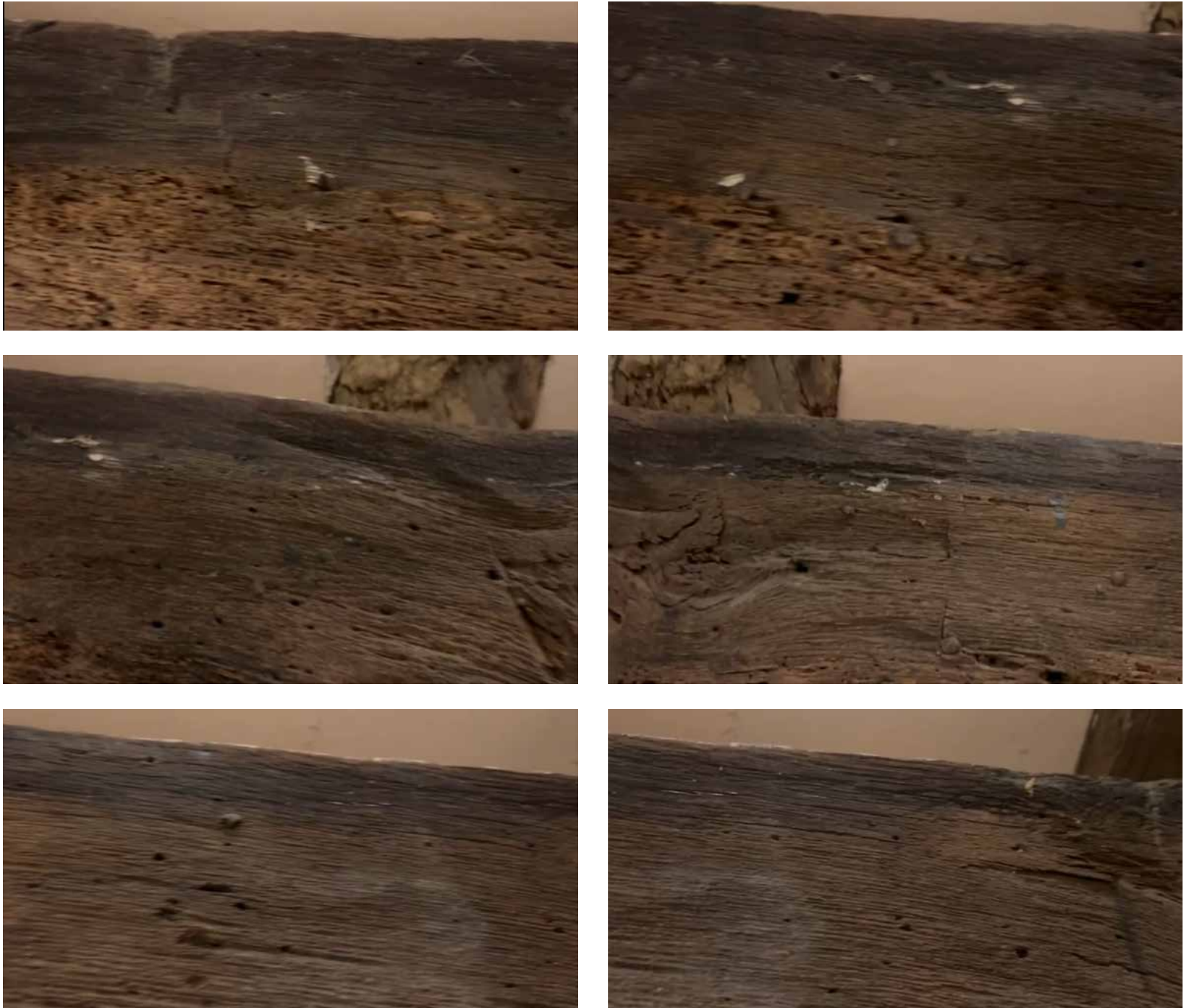
South bedroom timber frame photographs, November 2025
