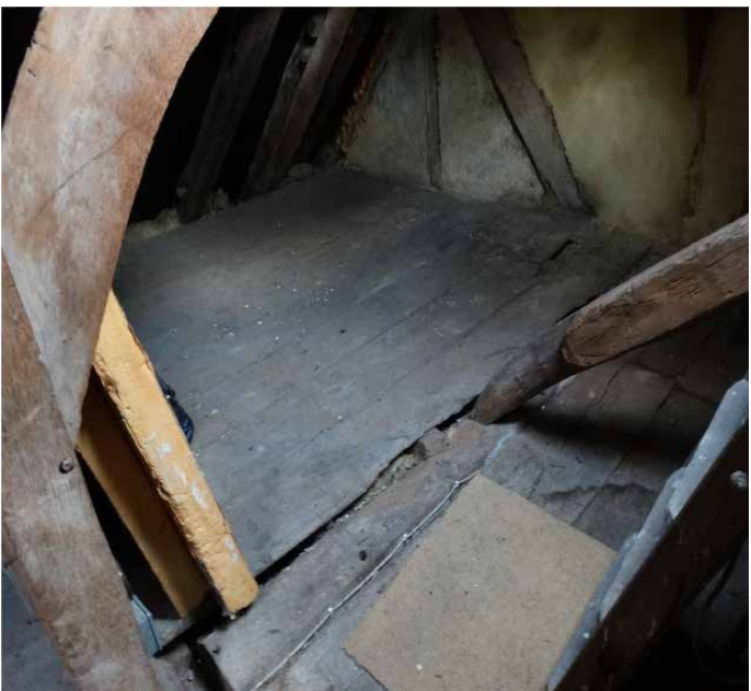
Extract from Desbrulais Heritage Report - area of attic floor with historic floorboards loose laid
